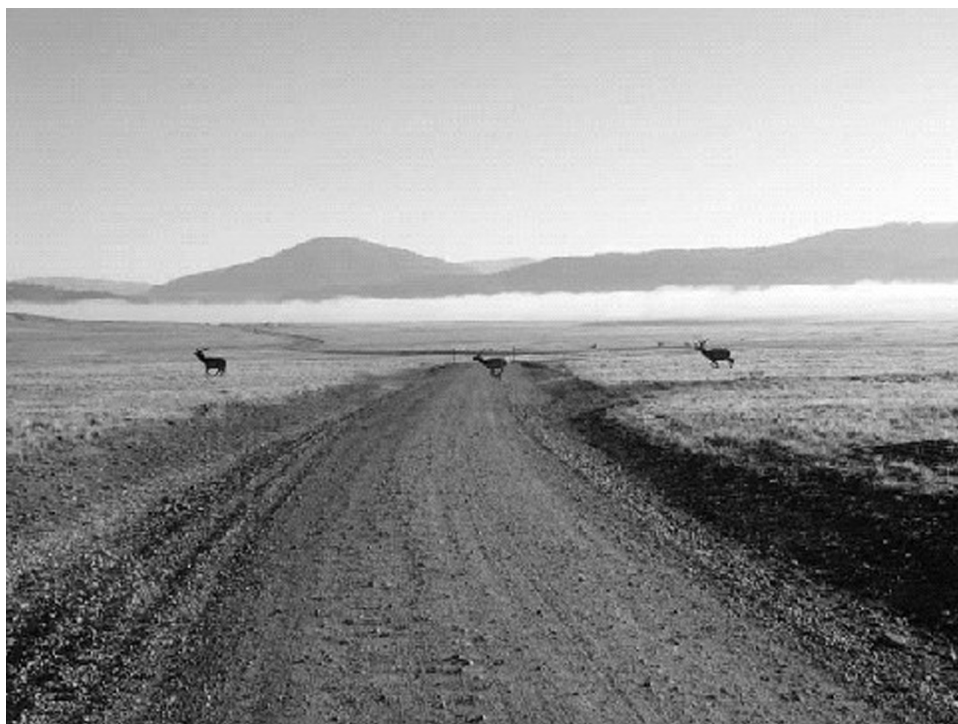
Figure 4: Portion of the Main Access Road to the Caldera after Rehabilitation
