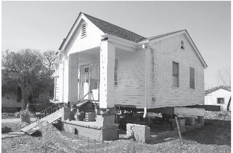
Figure 12: A New Orleans House Is Elevated Using ICC Coverage to Pay Some Costs
