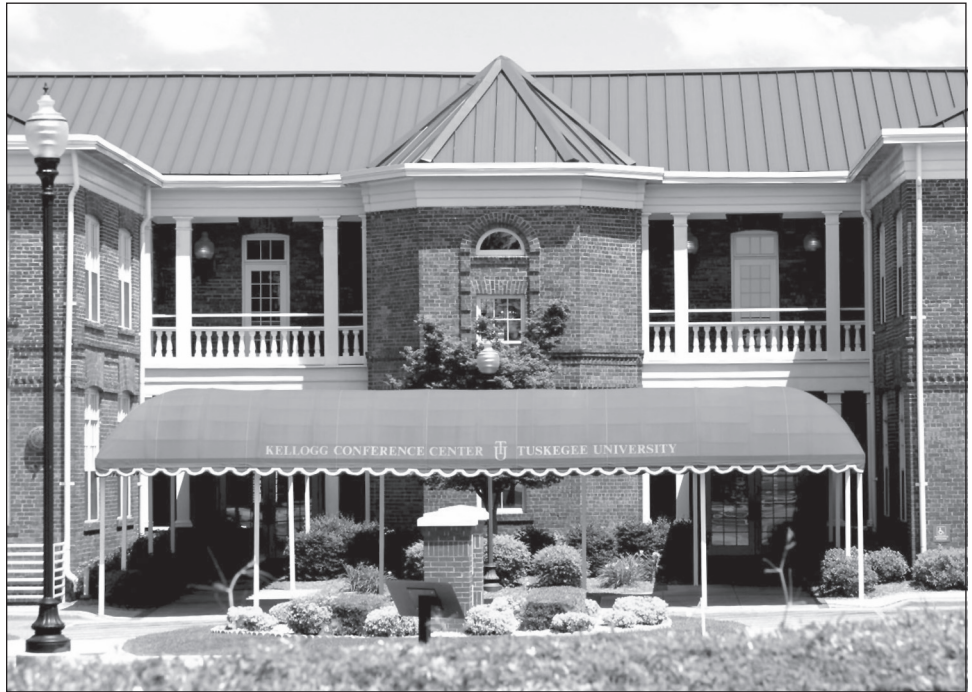
Figure 1: The Renovated Kellogg Conference Center at Tuskegee University
