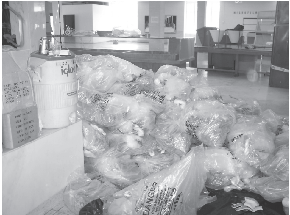
Figure 4: Removed Asbestos from Dillard University Library Awaiting Disposal
