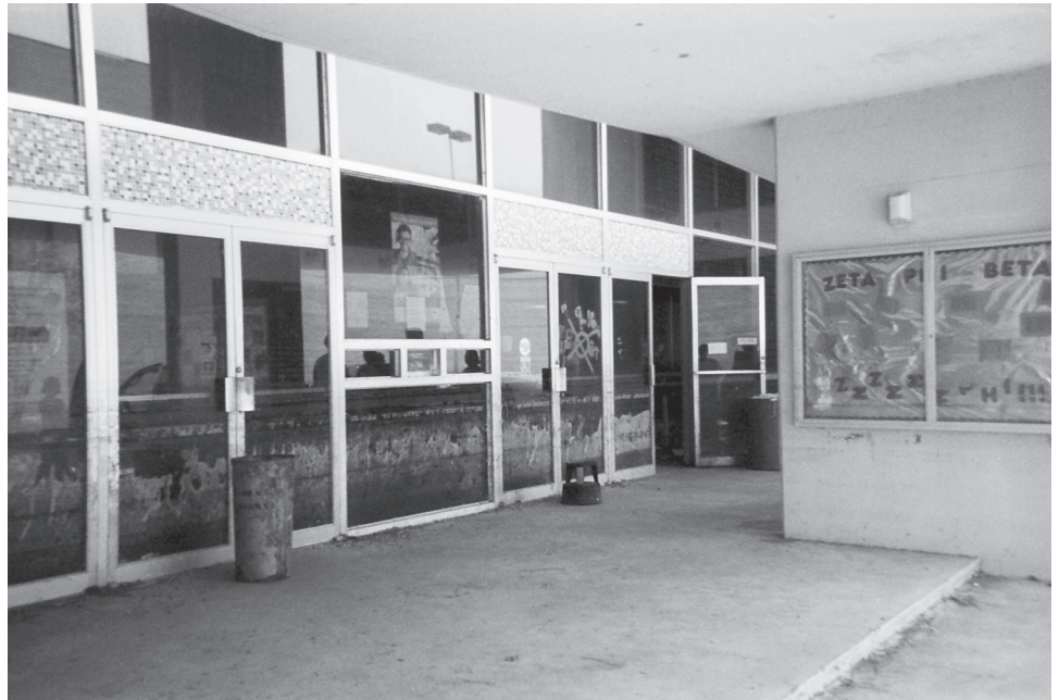
Figure 3: Exterior of Southern University's Library with Waterline Indicating the Extent of Flooding
