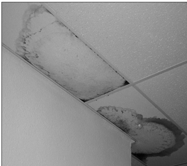
Roof Leaks
