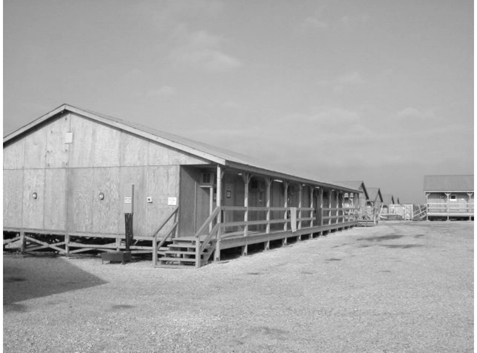
Figure 3: SEAhut in Kosovo With 100-Percent Power Redundancy
