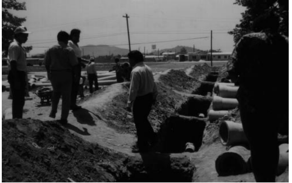
Figure 2.2: CARE Sewer Infrastructure Improvement Food-for-Work Project in Honduras
