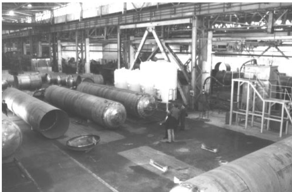
Figure I.2: Cryogenic Pressure Vessel Production at a Former Missile Production Facility
