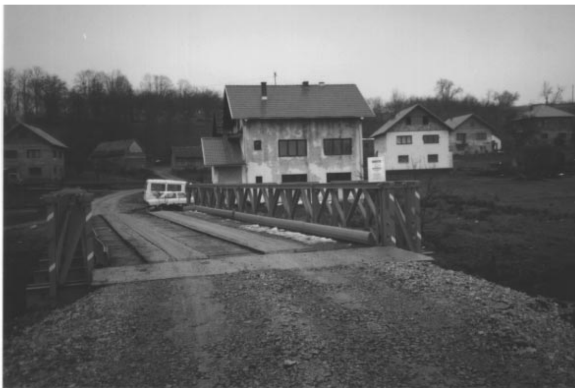
Figure 4.2: USAID-funded Housing and Bridge Repairs
