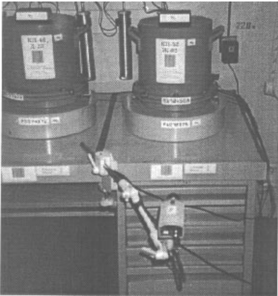
Cameras used to monitor nuclear material storage containers
