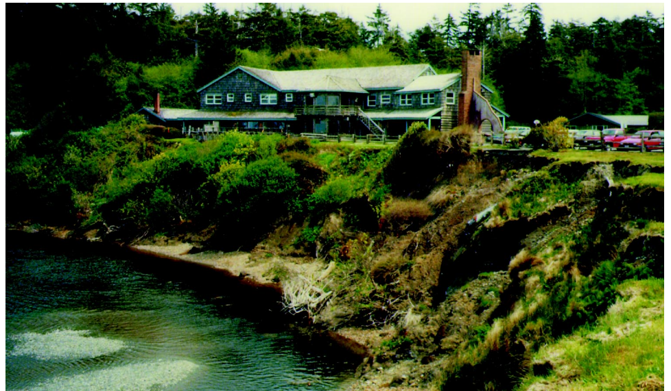
Figure 7: Condition of Cliff Near Kalaloch Lodge in Olympic National Park
