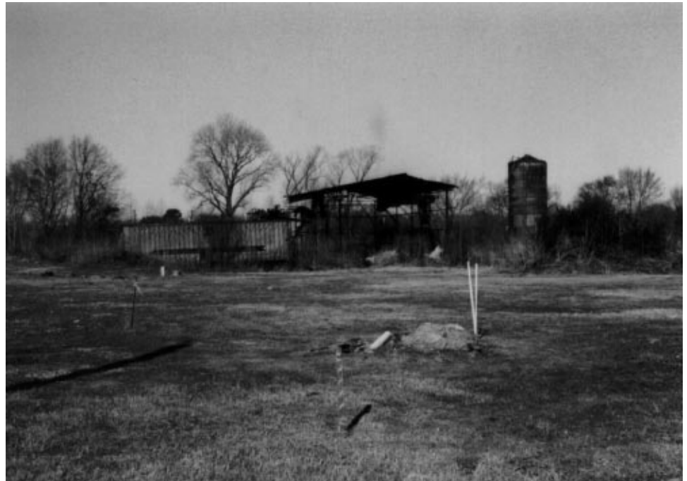
Figure I.1: Remaining Structures of the Wood Treating Operations at Texarkana
