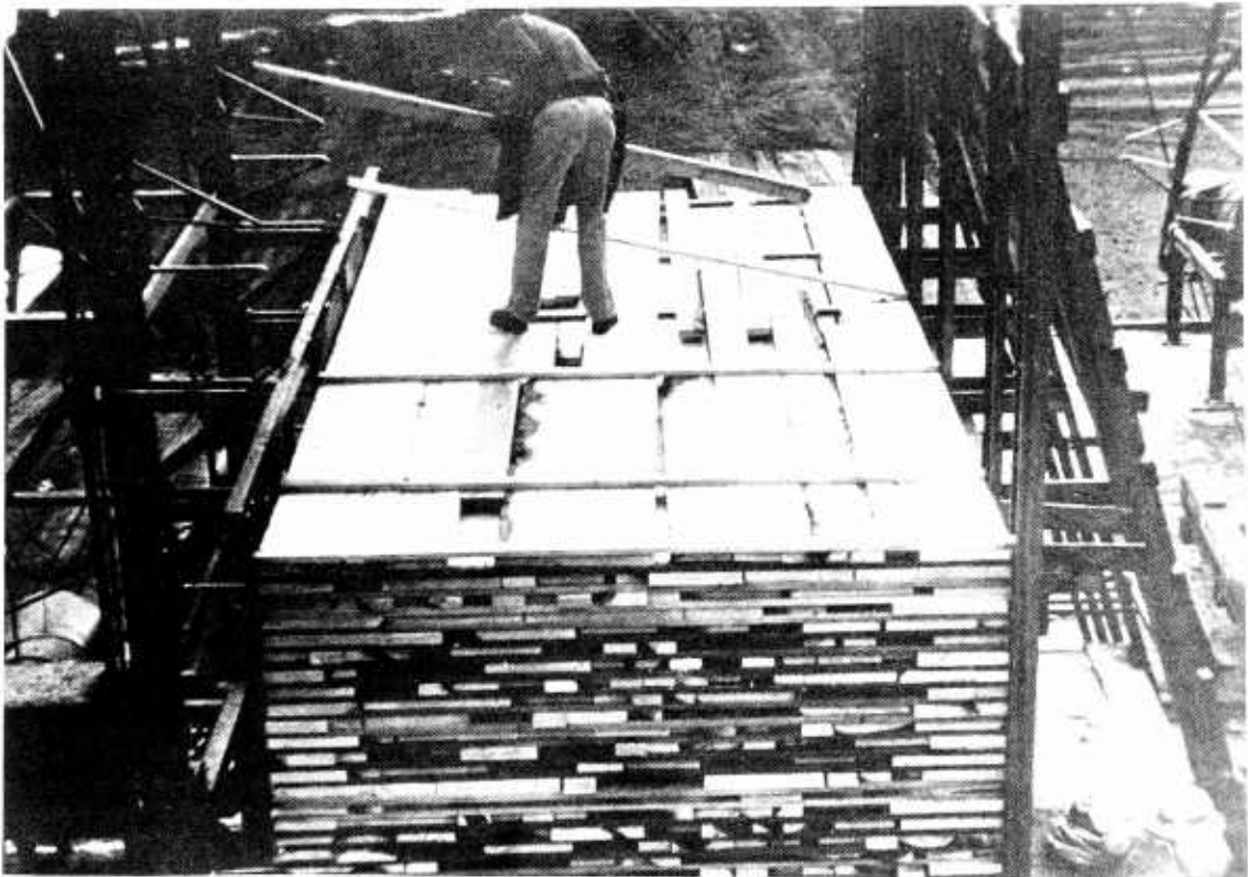
FIGURE 81.—Method II box piling, used for lumber of random length and width.
