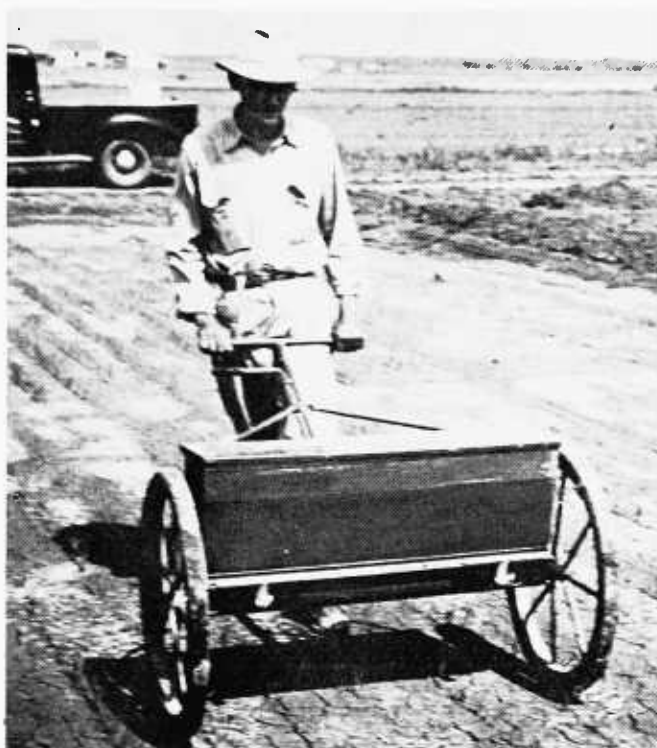
FIGURE 12.—A force-feed fertilizer used to distribute nitrogen as a topdressing.
