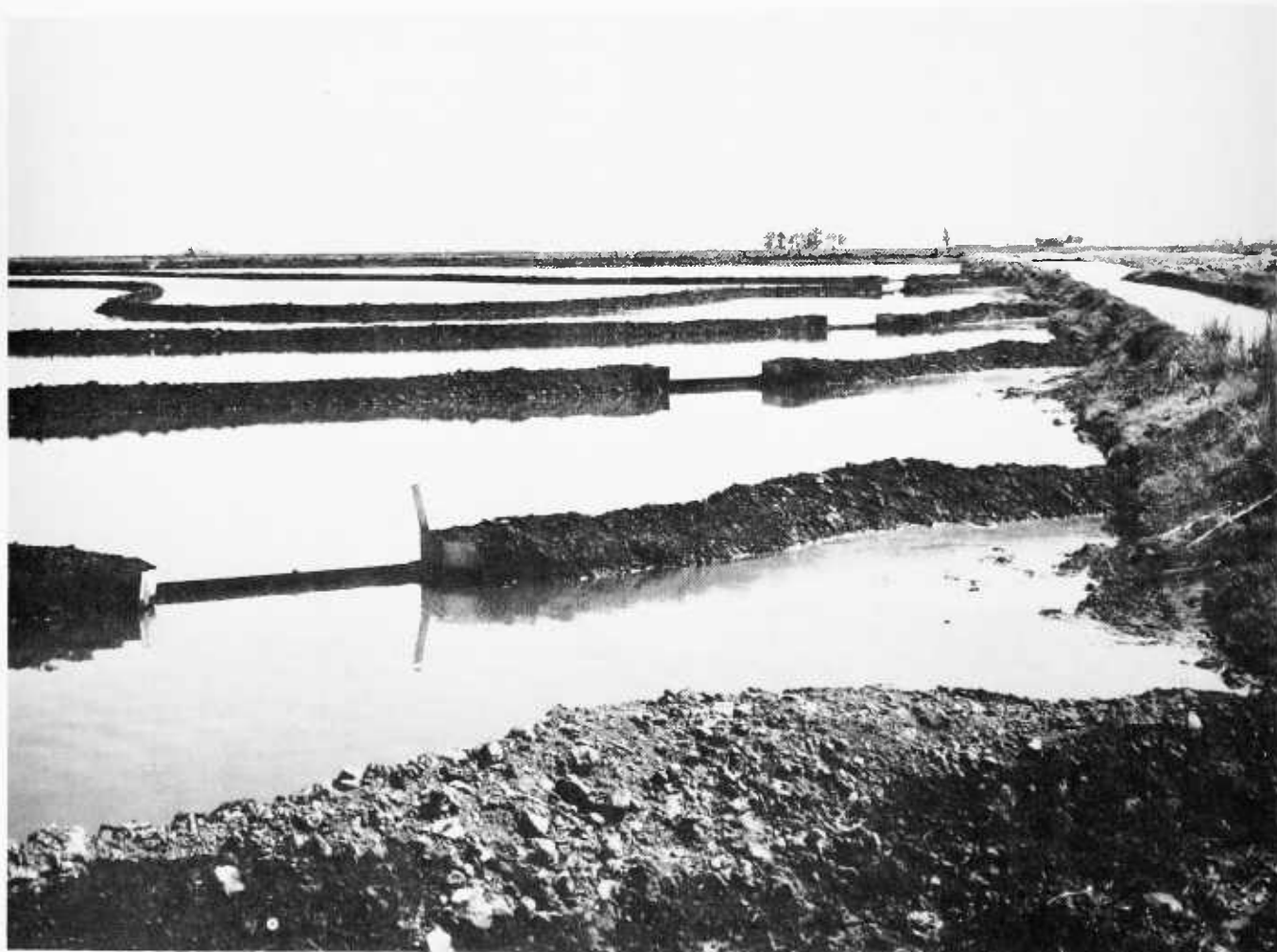
FIGURE 35.—A ricefield in Arkansas that is irrigated and ready to be seeded, showing the gates used to regulate the flow of water from one check to another. (Photo by Copeland.)
