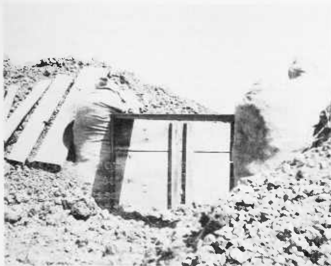
FIGURE 36.—Levee box used in California to regulate flow of water from one check to another in ricefield.
