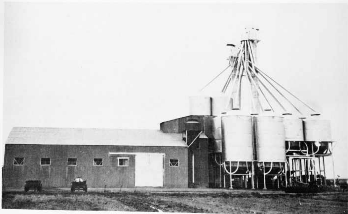
FIGURE 27.—Rice seed processing plant at Stuttgart, Ark.
