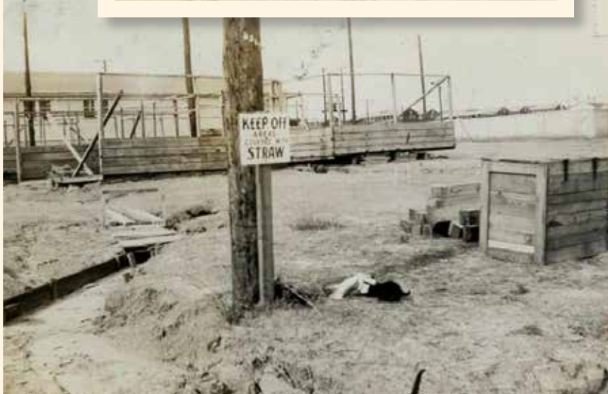
Pyramidal-type tent frames under construction.
