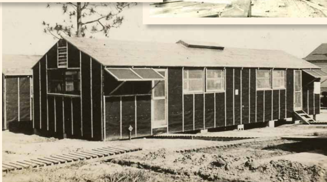
Hutments are completed with screens and roof ventilation.
