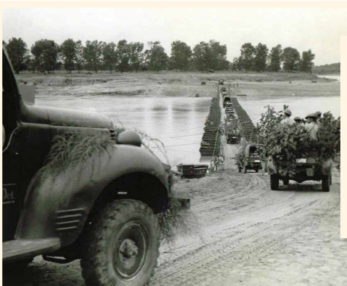
A 367-foot bridge across the Sabine River built in 5 hours by Company A, 7 th Engineers.
