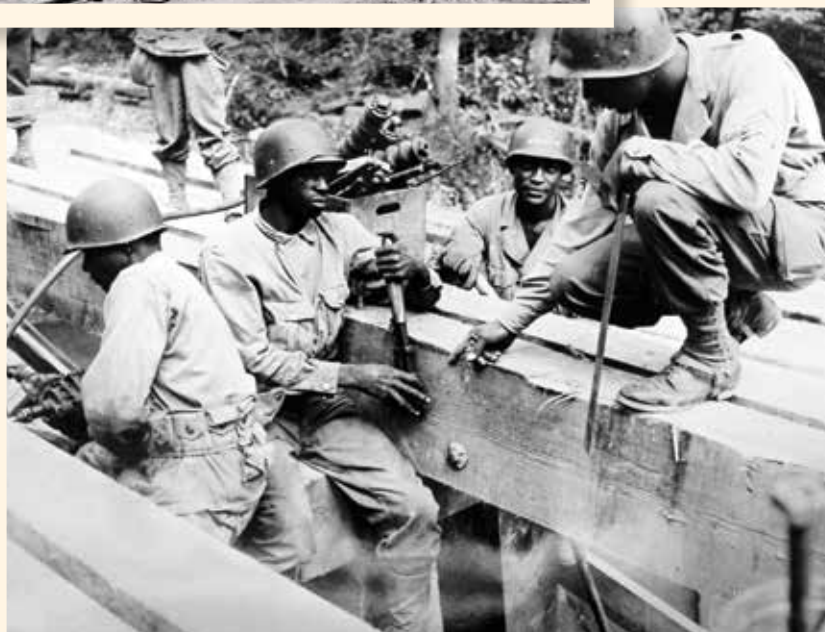
EUTC engineers constructing a wooden bridge on the Claiborne-Polk Railroad.
