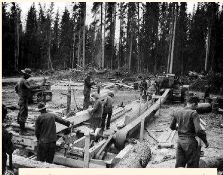
Typical portable sawmill used by Engineer Forestry Battalions.
