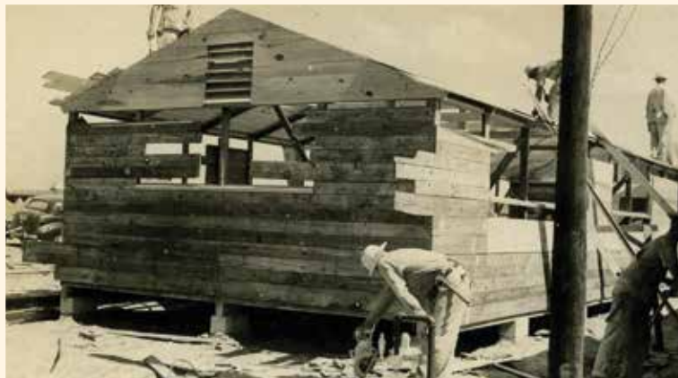
The roof and wood siding is installed on a hutment.
