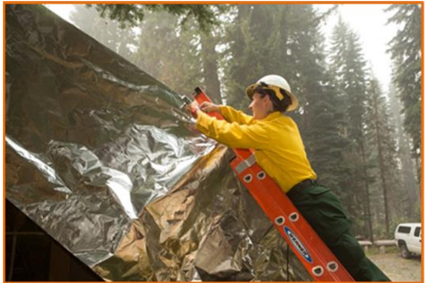
A member of the Columbia River Fire Crew wraps a structure in the Cottonwood Guard Station to protect it from the approaching Wolverine Fire. Photo by Kari Greer, U.S. Forest Service.
