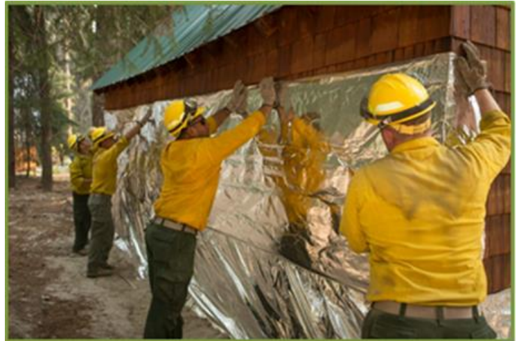
Washington National Guard firefighters wrap cabins in the Pope Creek area in the Entiat Valley on the Wolverine Fire. Photo by Kari Greer, U.S. Forest Service.
