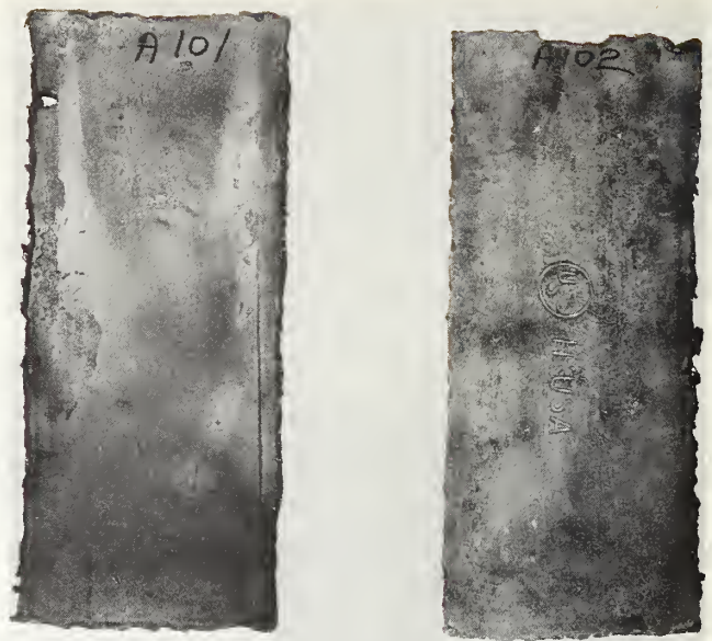
FIGURE 5. Steel sheet piling sections (2 ft by 1 ft) cut from two locations on the Memphis Floodwall after exposure for 6.3 years.
