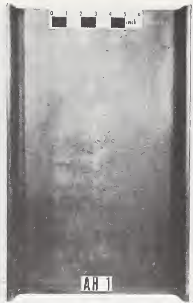
FIGURE 2 – Section of steel I-beam pulled from a pier on Lake Ontario at Olcott, N. Y., after exposure for 50 years. The section was exposed about 2 ft below the mud line and was practically unaffected by corrosion.
