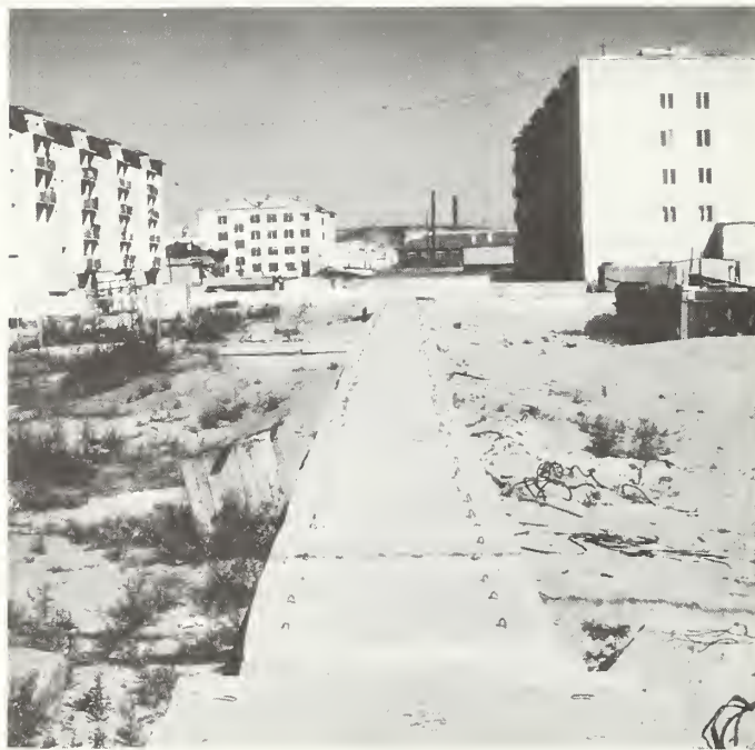
Figure 14 Precast concrete utilidor in Yakutsk, USSR.
