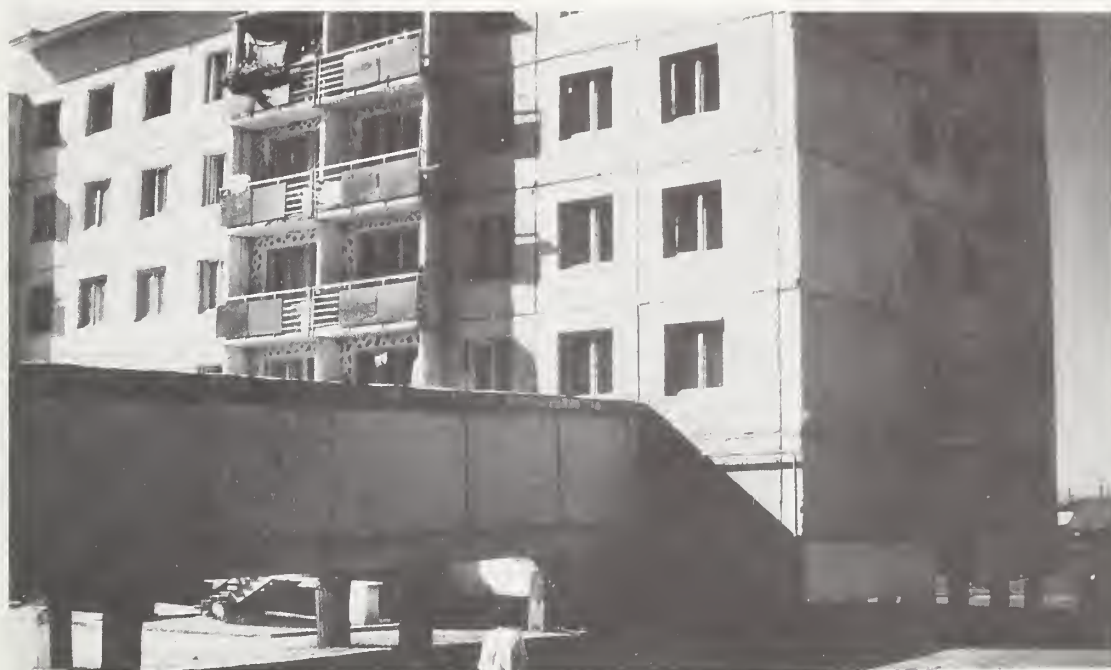
Figure 15 An elevated utilidor constructed on piles between apartment buildings in Yakutsk, USSR.
