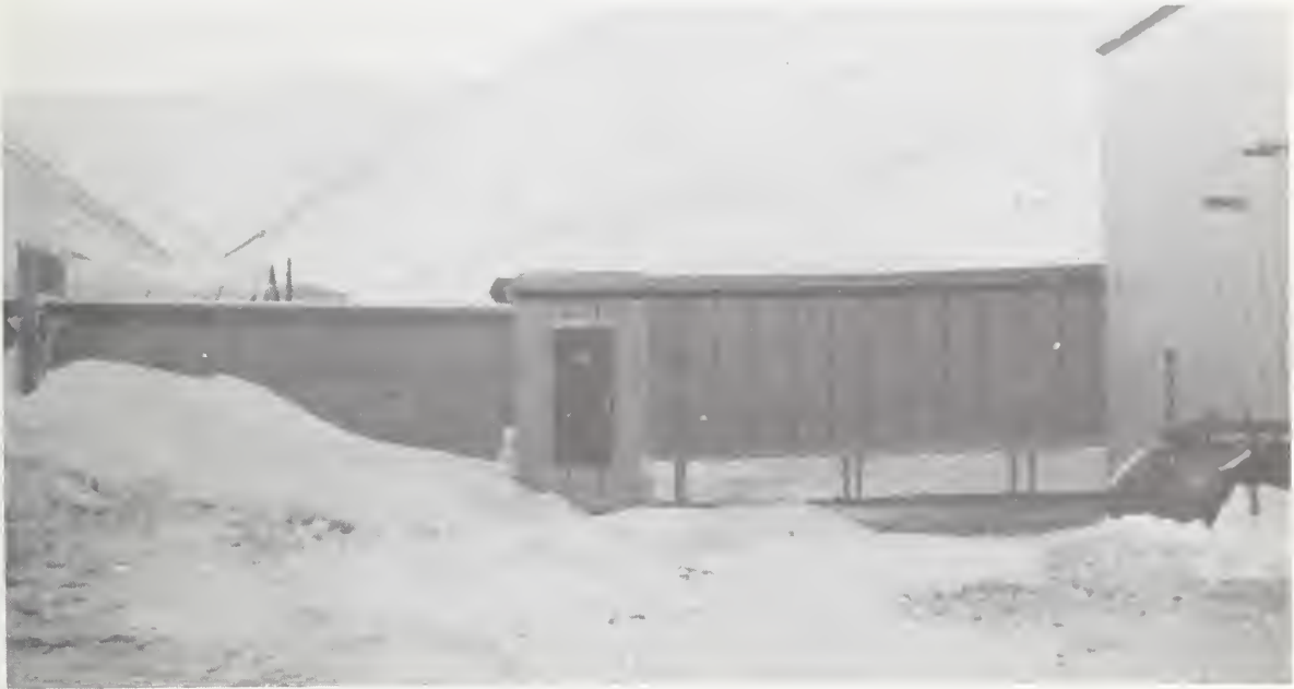
Figure 7 Variation in snow drifting in the lee of on-grade and elevated sections of the walkway-utilidor at Cape Lisburne, Alaska.
