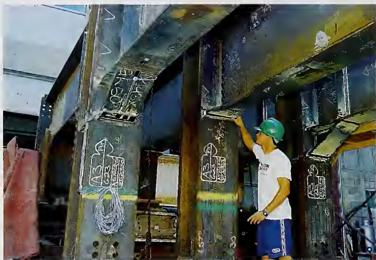
Investigation of beam column connections
