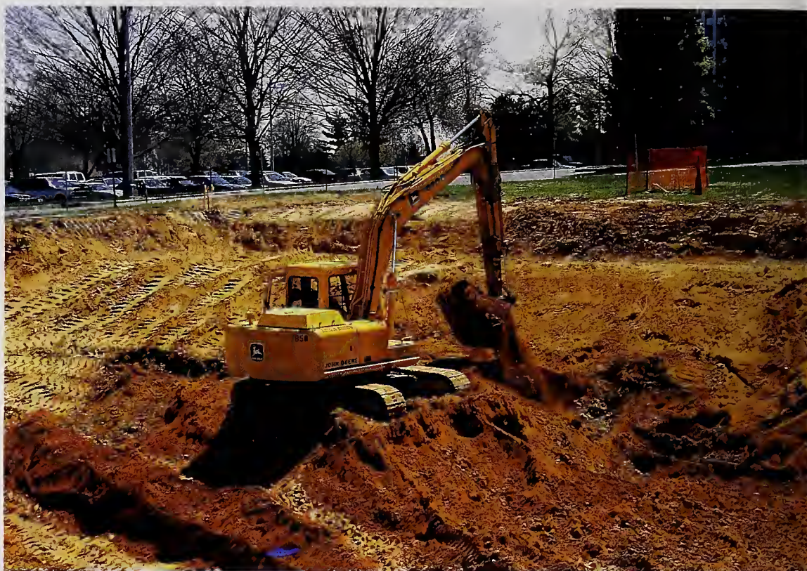
Excavation for NIST's new Advanced Chemical Sciences Laboratory
