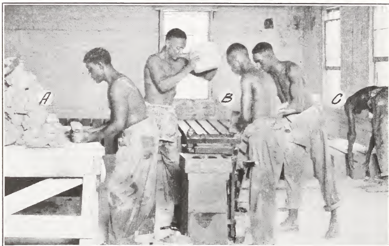
FIG. 14.— Forming of brick by hand
