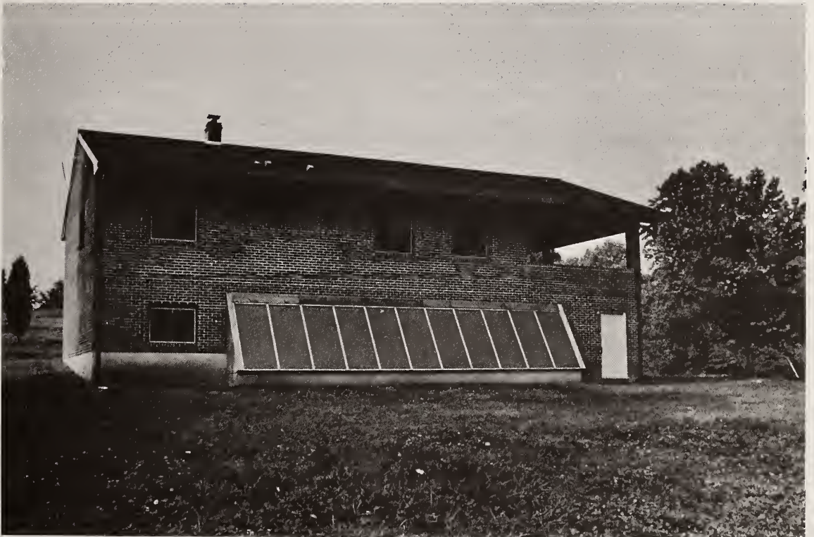
Figure 7 - South Face of Split Foyer Home
