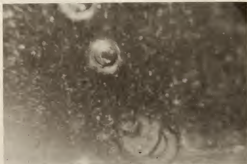
Figure 7. Photographs of corrosion of the samples corresponding to the results presented in figure 6.
