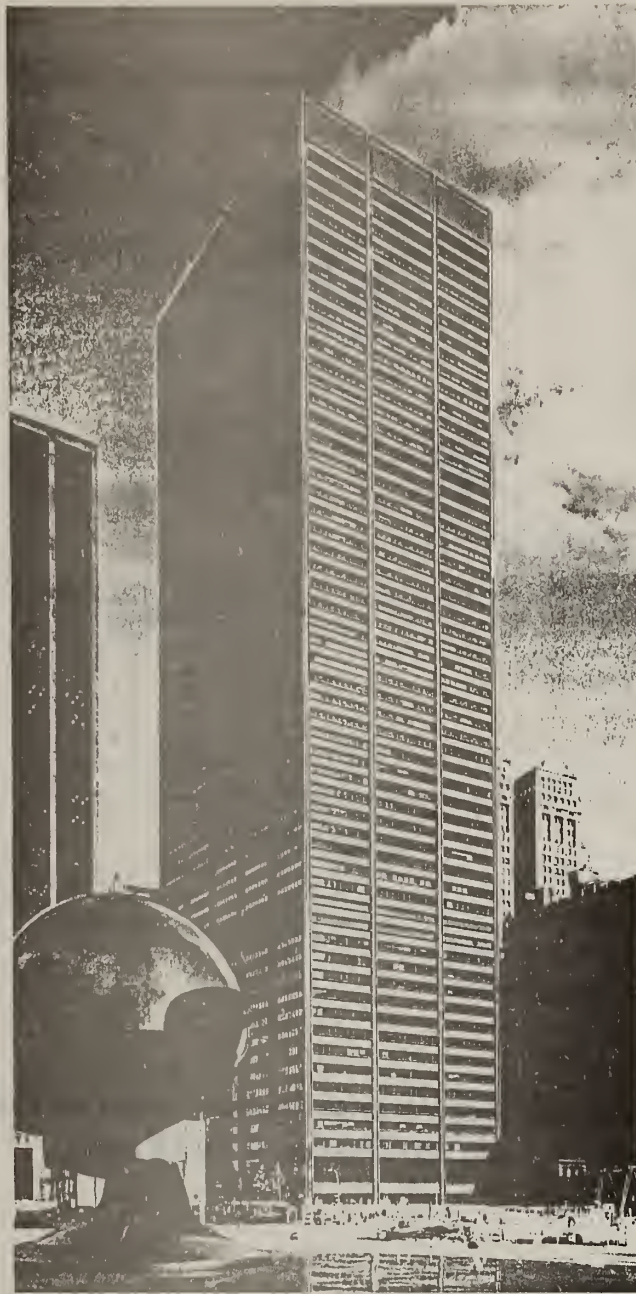
Figure 2 -- One Liberty Plaza, N.Y.C., exterior surfaces of steel spandrel beams have the web bare and the flanges flame-shielded.
