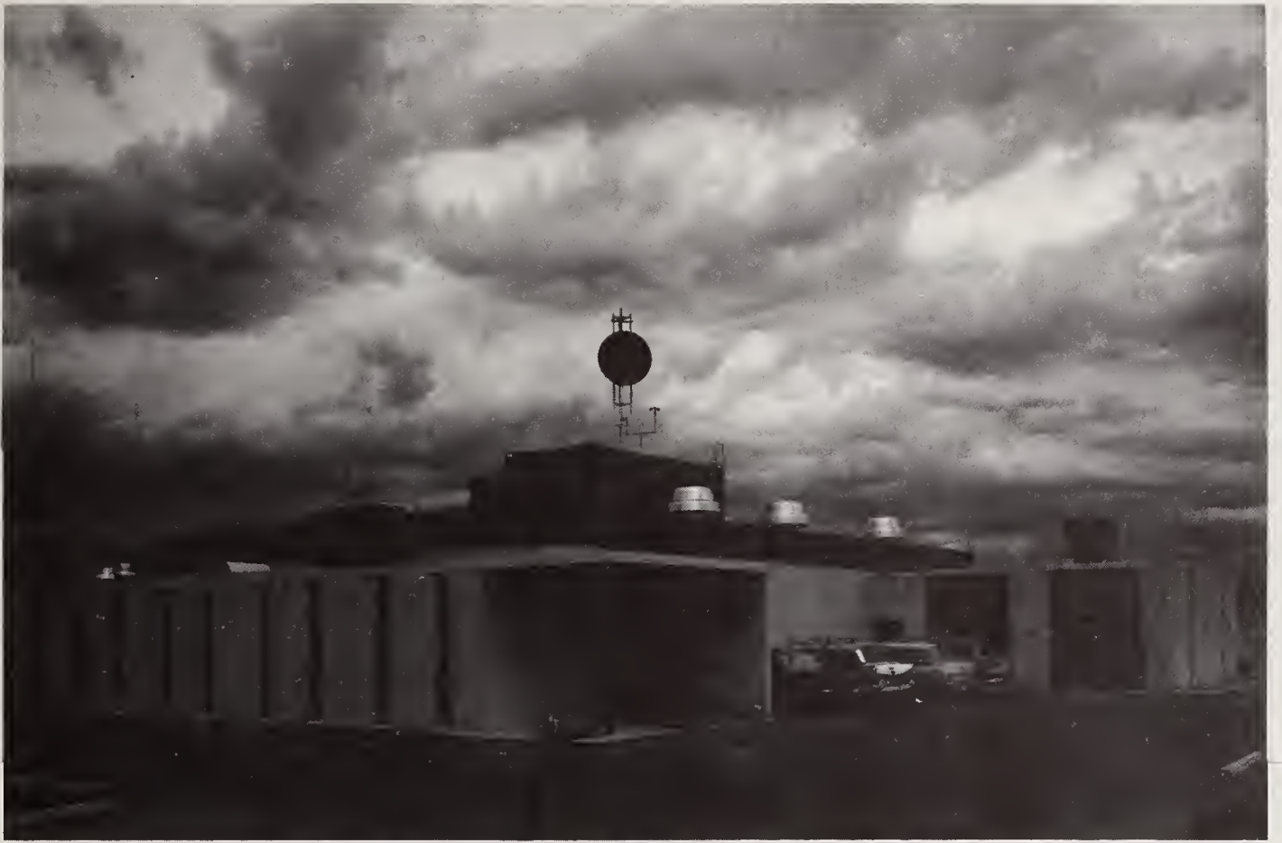
NBS Fort Collins facility showing WWV transmitter building.
