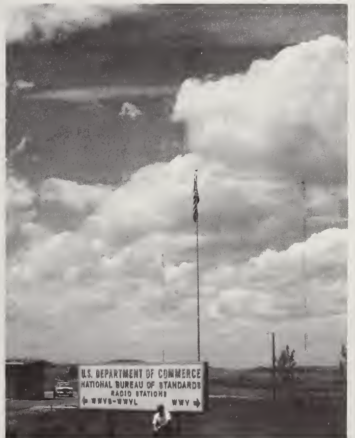
WWVB/WWVL transmitter building and antennas.
