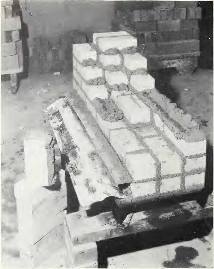
FIGURE 8.—Brick wall of workmanship A'.
