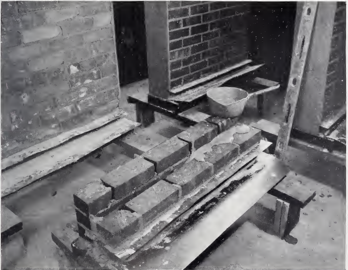
FIGURE 11.—Brick wall of workmanship H, grouted.
