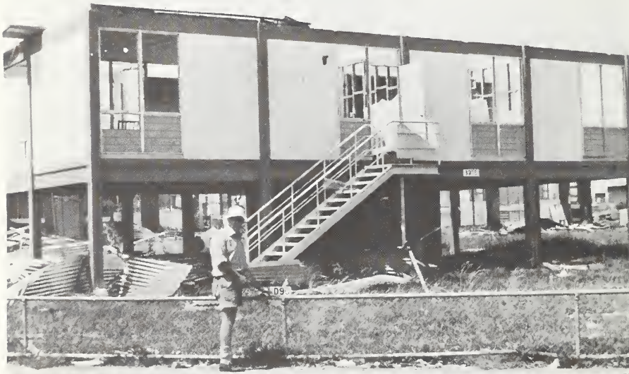
Fig. 12. High-set house with precast concrete frame and interlocking precast concrete panels.
