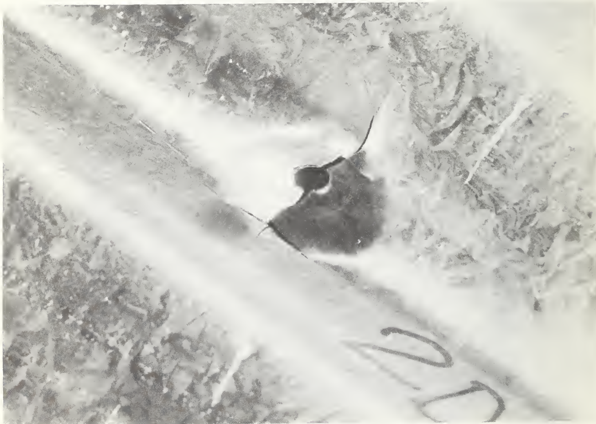
Fig. 32. Typical fatigue failure of CGI cladding
