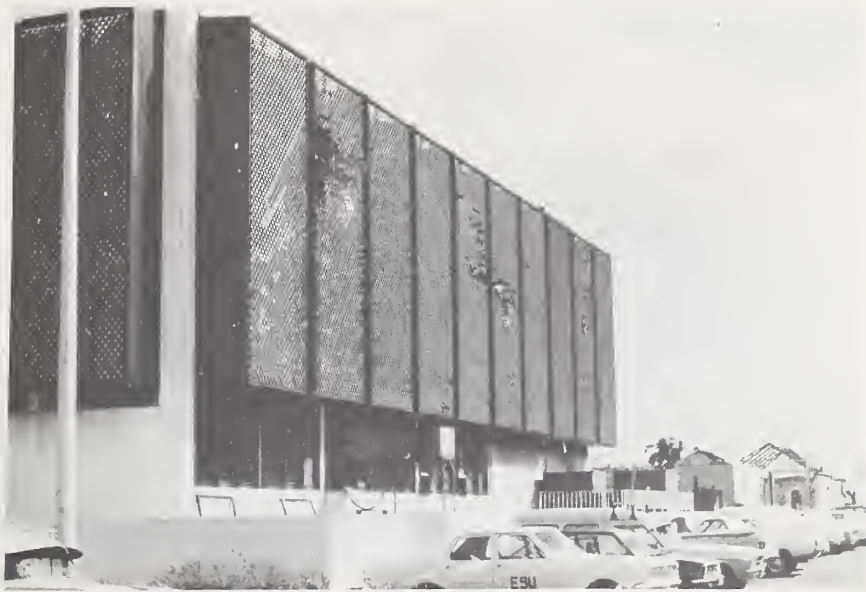
Fig. 25. Sunscreen showing points of missile impact
