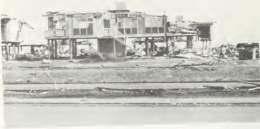
Fig. 3. Typical high-set house
