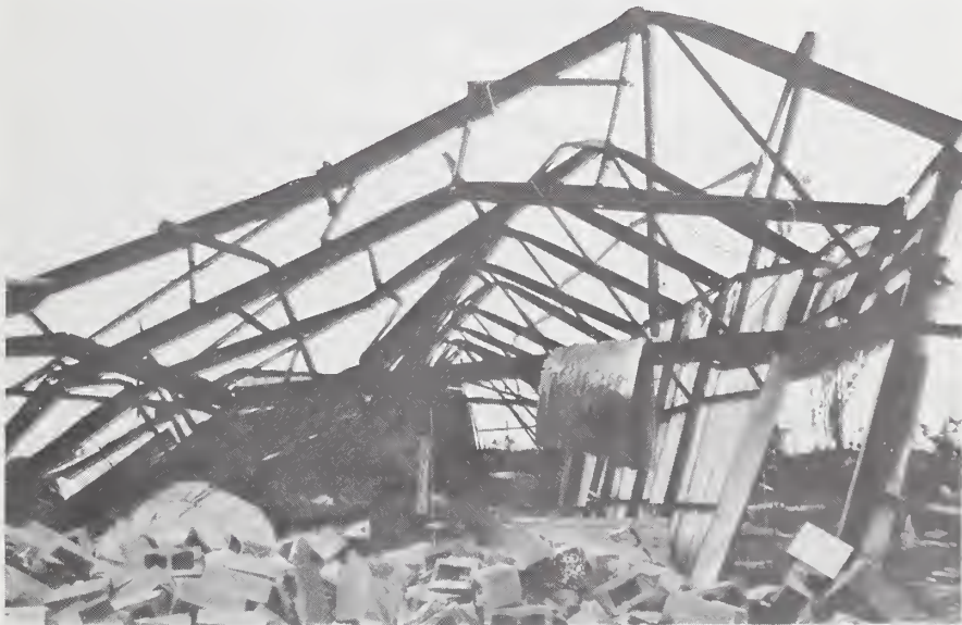
Fig. 30. Industrial building - Winnellie
