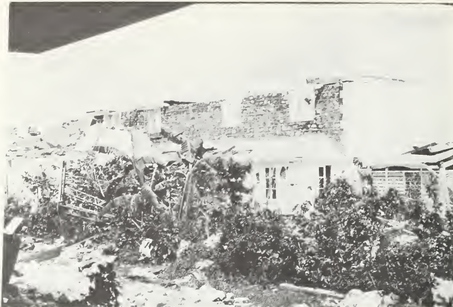
Fig. 27. Historic building in Darwin City - hip roof completely removed
