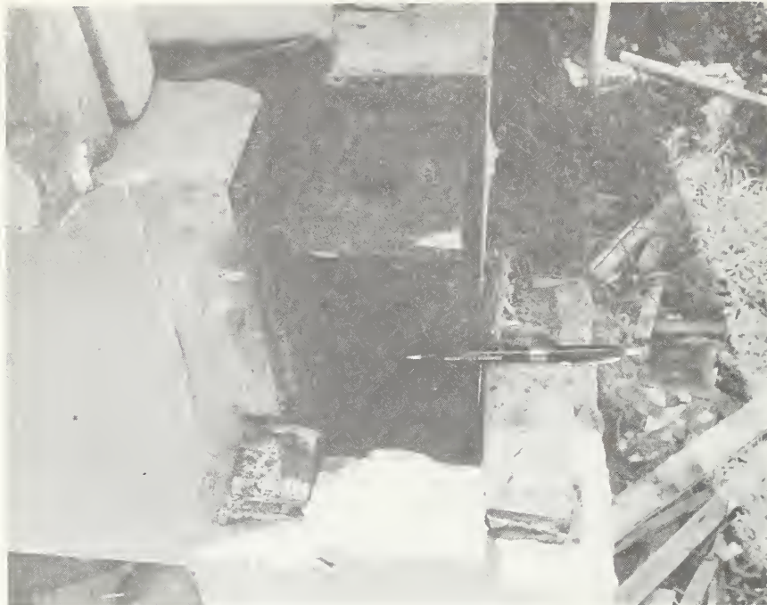
Fig. 15. Beam to column connection - precast concrete high-set
