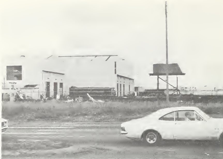
Fig. 31. Railway shops - Stuart Park
