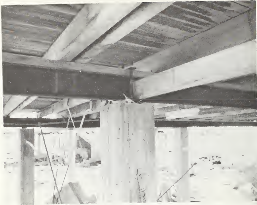
Fig. 7. Typical floor systems and pier anchorage
