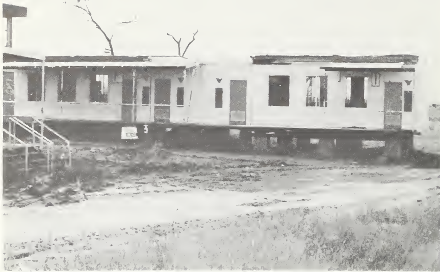
Fig. 19. Temporary classrooms - Millner Primary School
