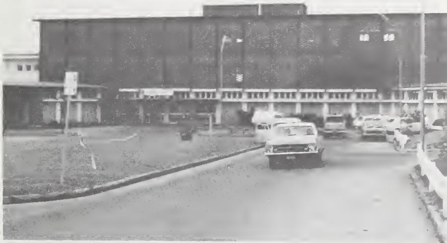
Fig. 26. Darwin Hospital - Larrakeyah
