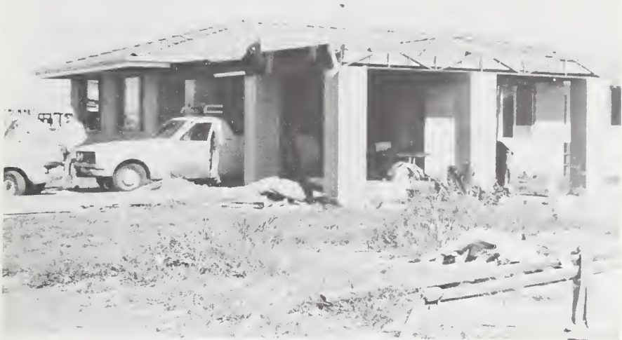
Fig. 17. Privately constructed residence with welded steel frame and brick veneer
