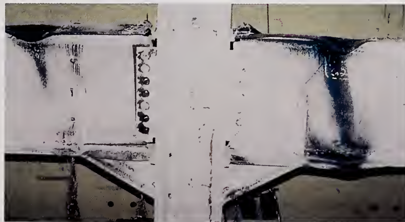
Experimental investigation of welded haunched retrofit
