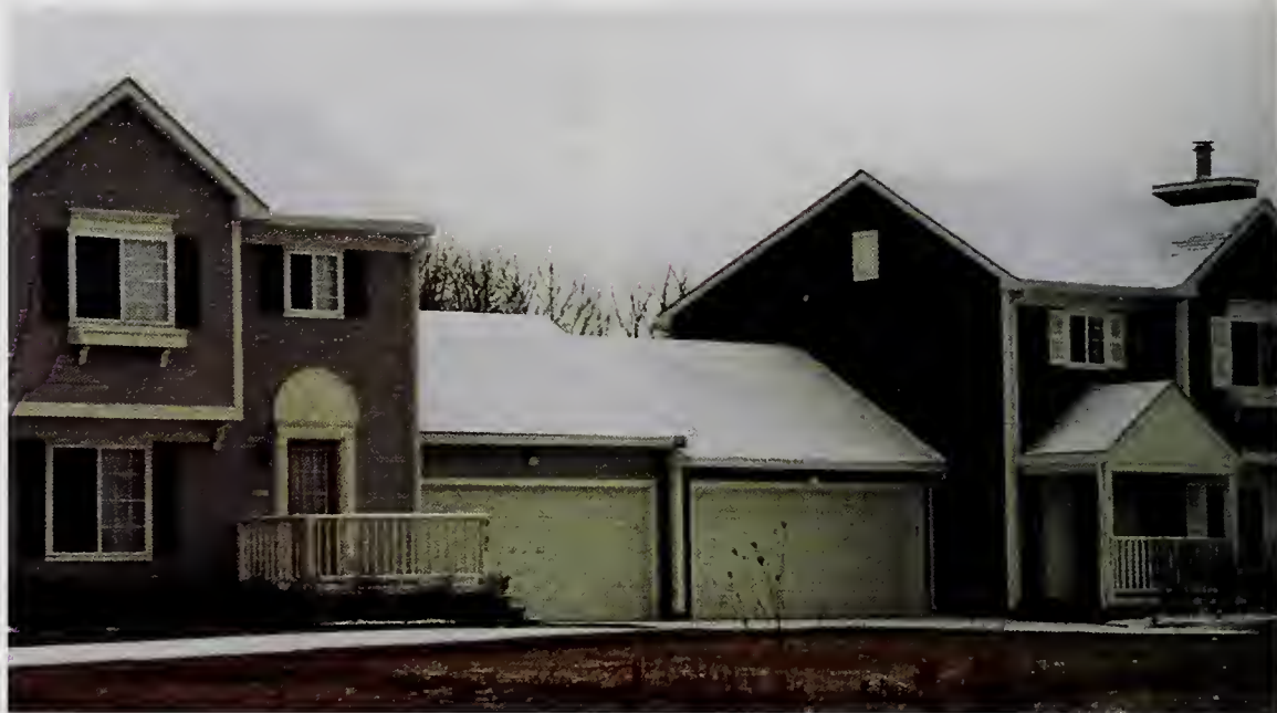
These superinsulated duplexes look normal but they use only half the space heating energy of conventional houses, saving their owners about $200 each year
