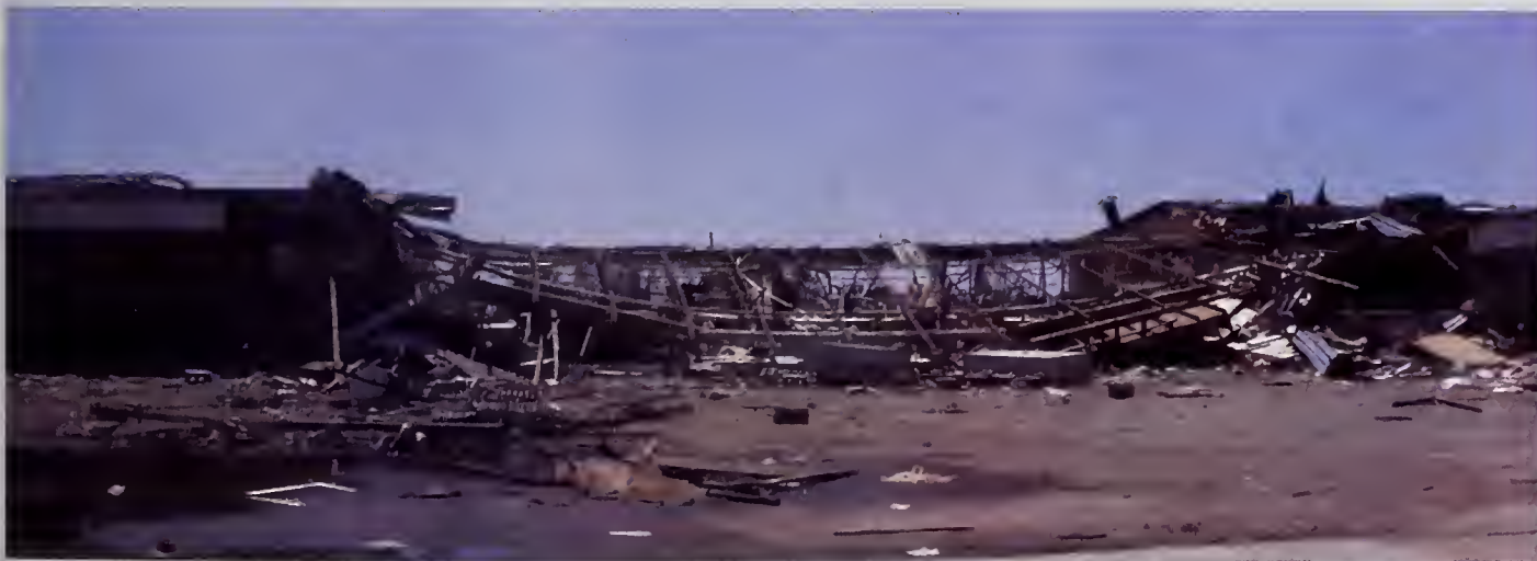
Kelley Elementary School in Moore, Oklahoma was destroyed by a direct hit from an F-5 rated tornado.
