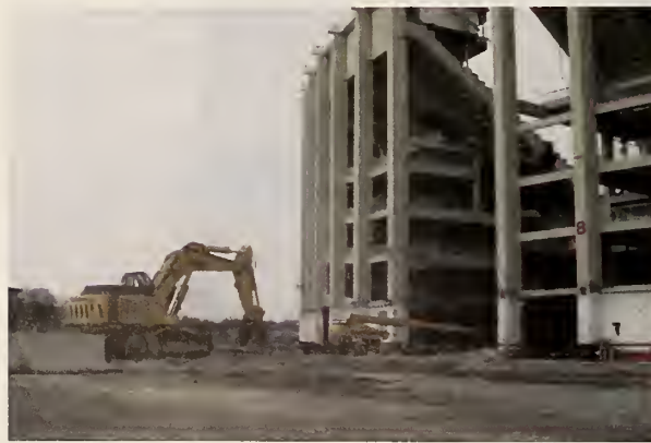
Figure 2. Pre-implosion deconstruction of the stadium.
