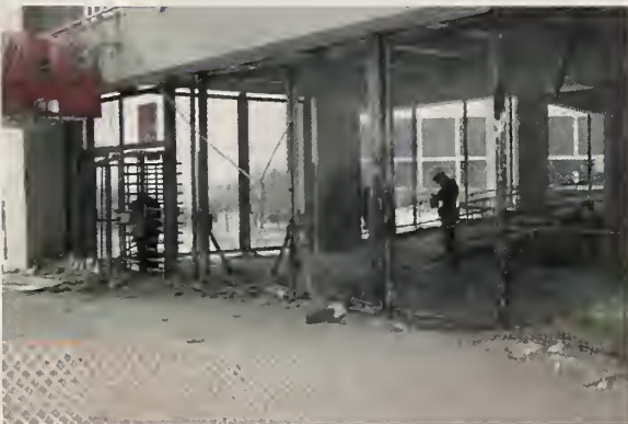
Figure 3. Pre-implosion preparation inside the stadium.
