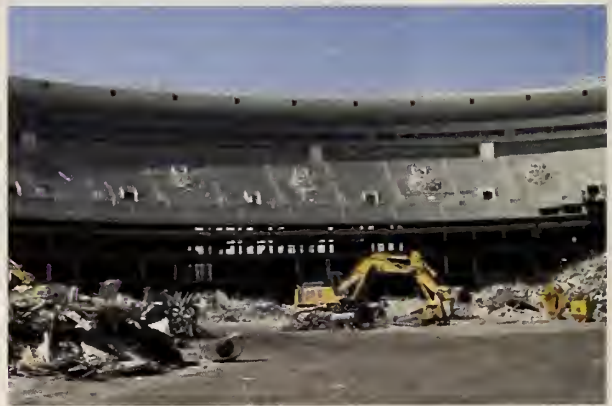
Figure 2. Pre-implosion deconstruction of the stadium.
