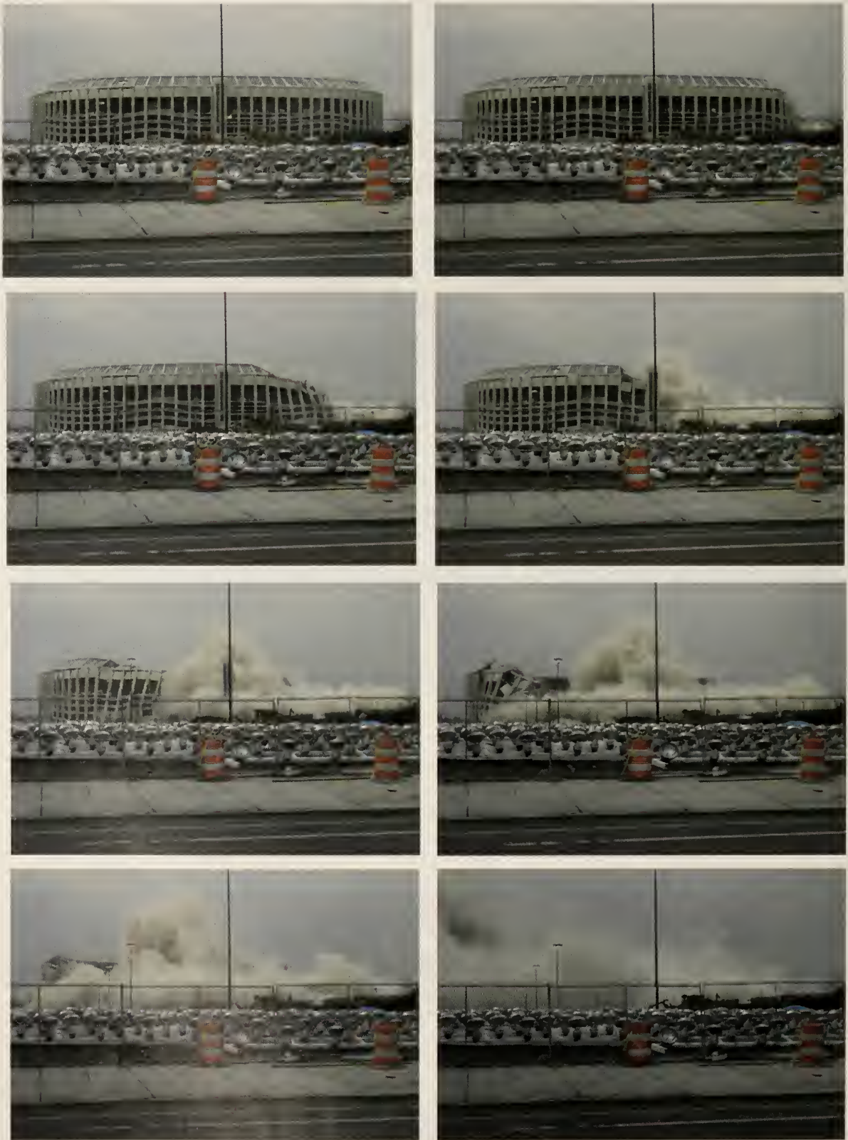
Figure 70. The stadium collapses during the implosion sequence.
