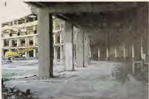
Figure 3. Pre-implosion preparation inside the stadium.
