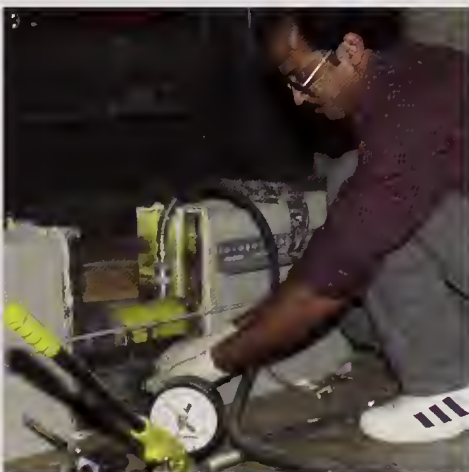
Bond strength test of glass fiber rods epoxied in mortar joints of concrete blocks.
