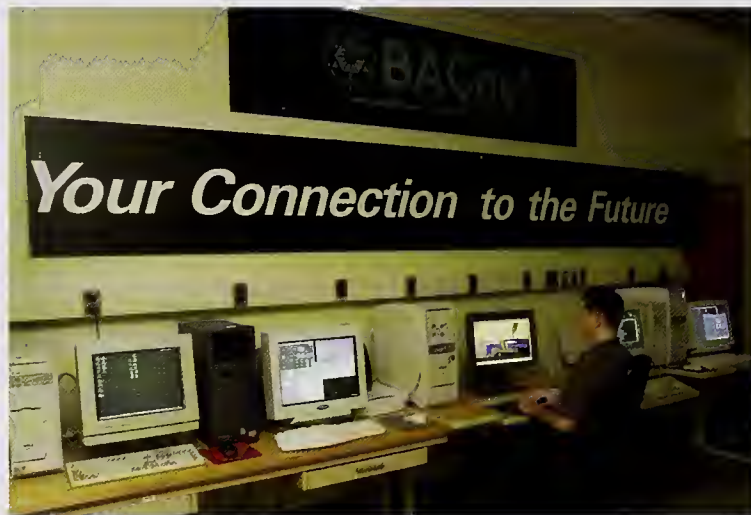
Virtual Cybernetic Building Testbed Control System Hardware.
