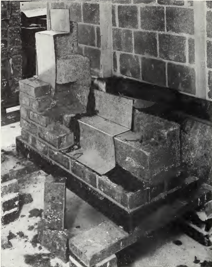
FIGURE 4.—Wall B236 during construction.
