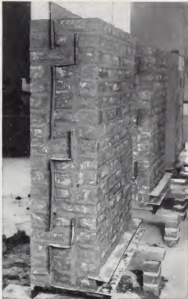
FIGURE 5.— Brick wall containing membrane waterproofing.
