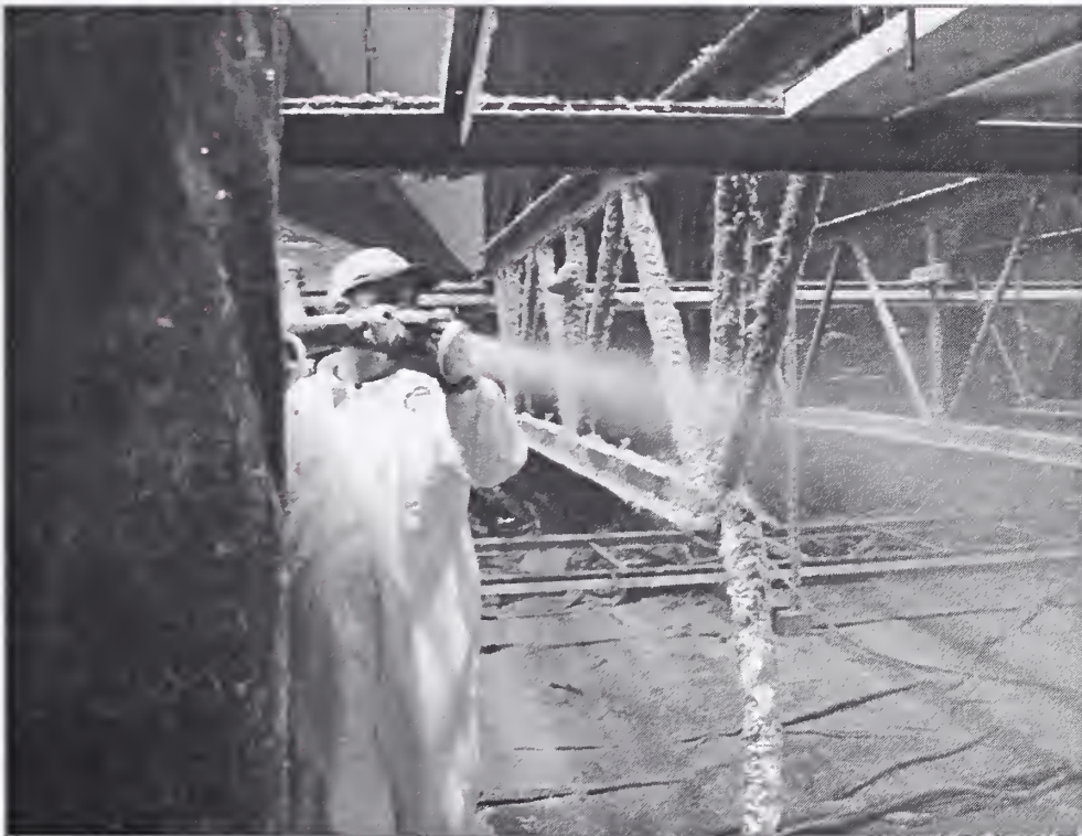
Figure 9-6d. Application of SFRM product to a truss.
