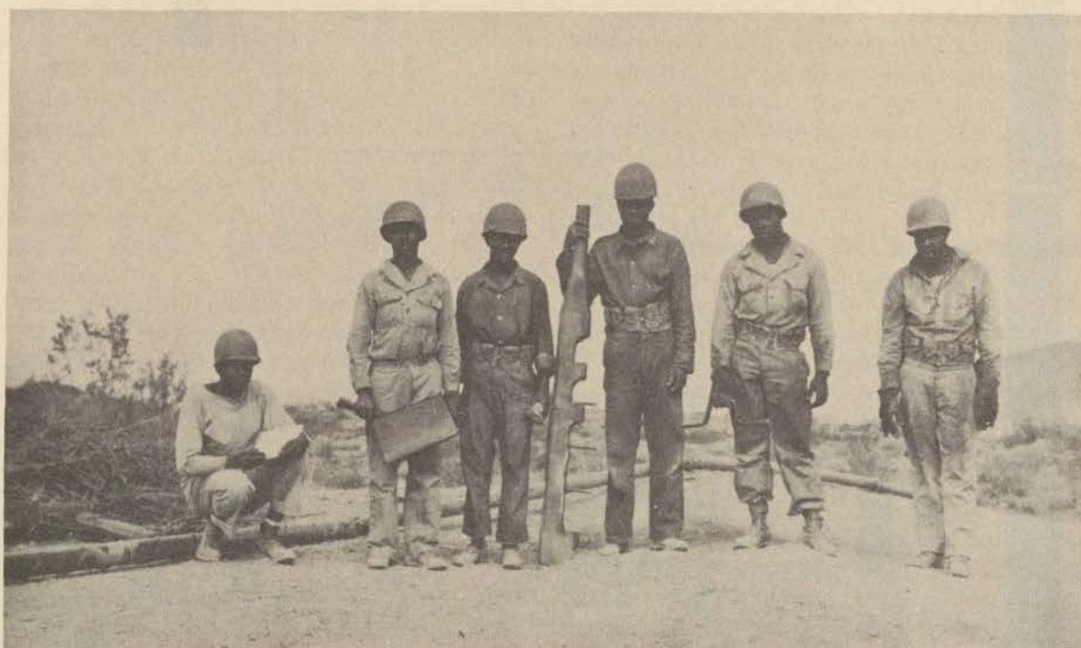
Figure 49. Coupling crew holding lazy board, jack, and speed wrench.
