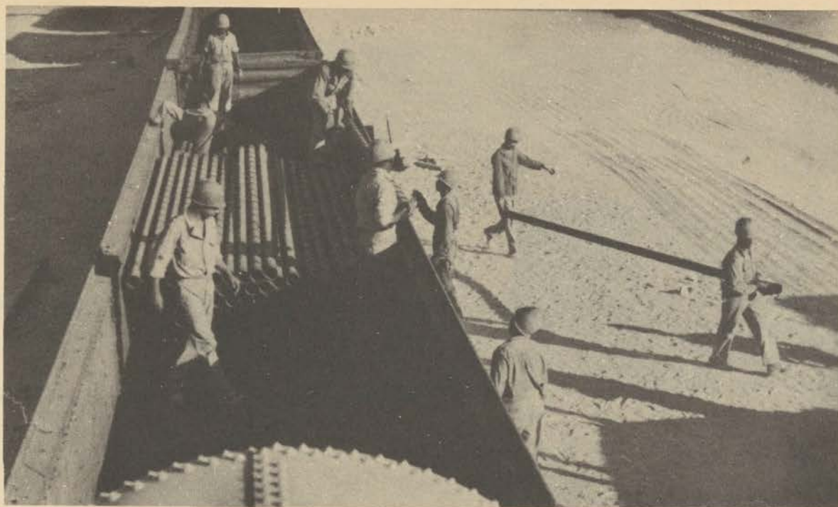
Figure 40. Unloading 4-inch spiral-weld pipe.
