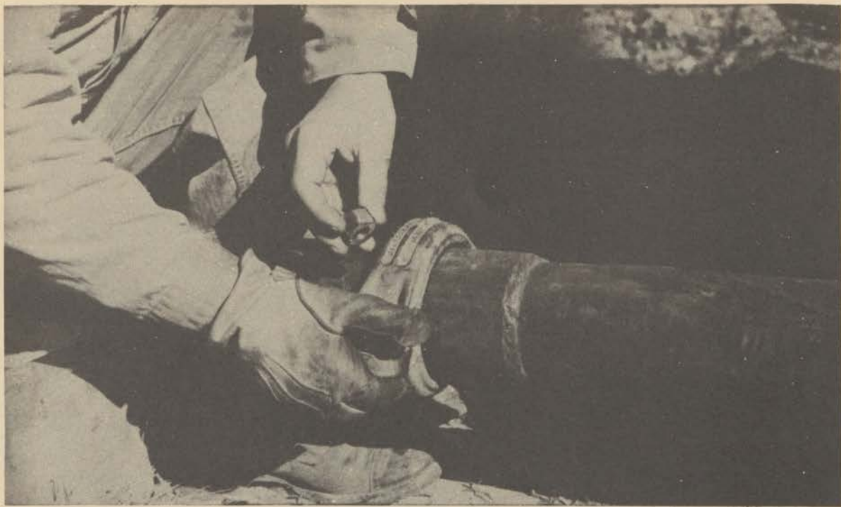
Figure 56. Holding coupling in place while bolting it together.
