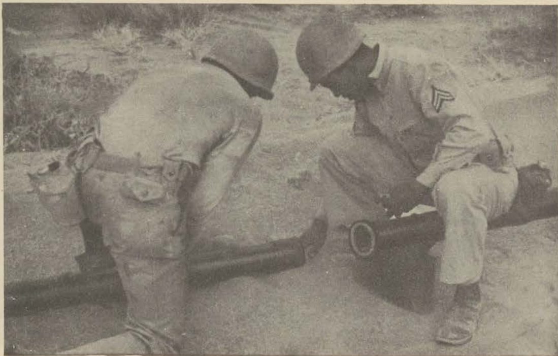
Figure 53. Preparing pipe joint for alinement. The end of the assembled pipe line is on the lazy board.
