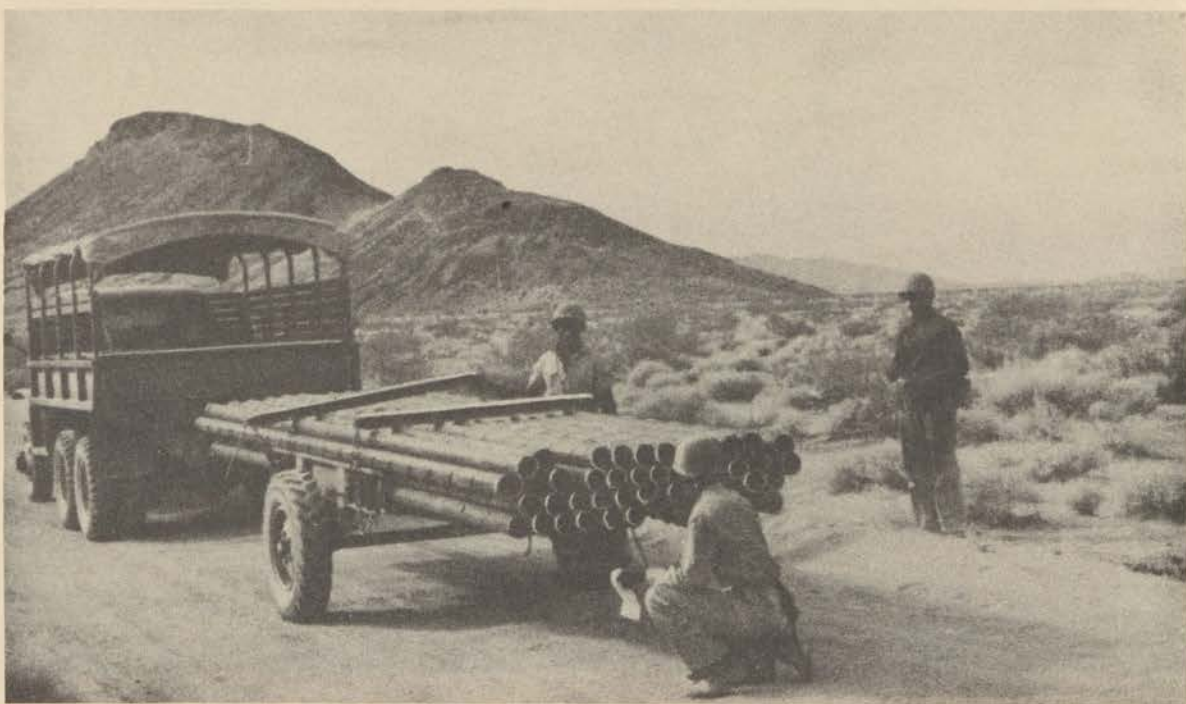
Figure 43. Removing booms during pipe string operation.
