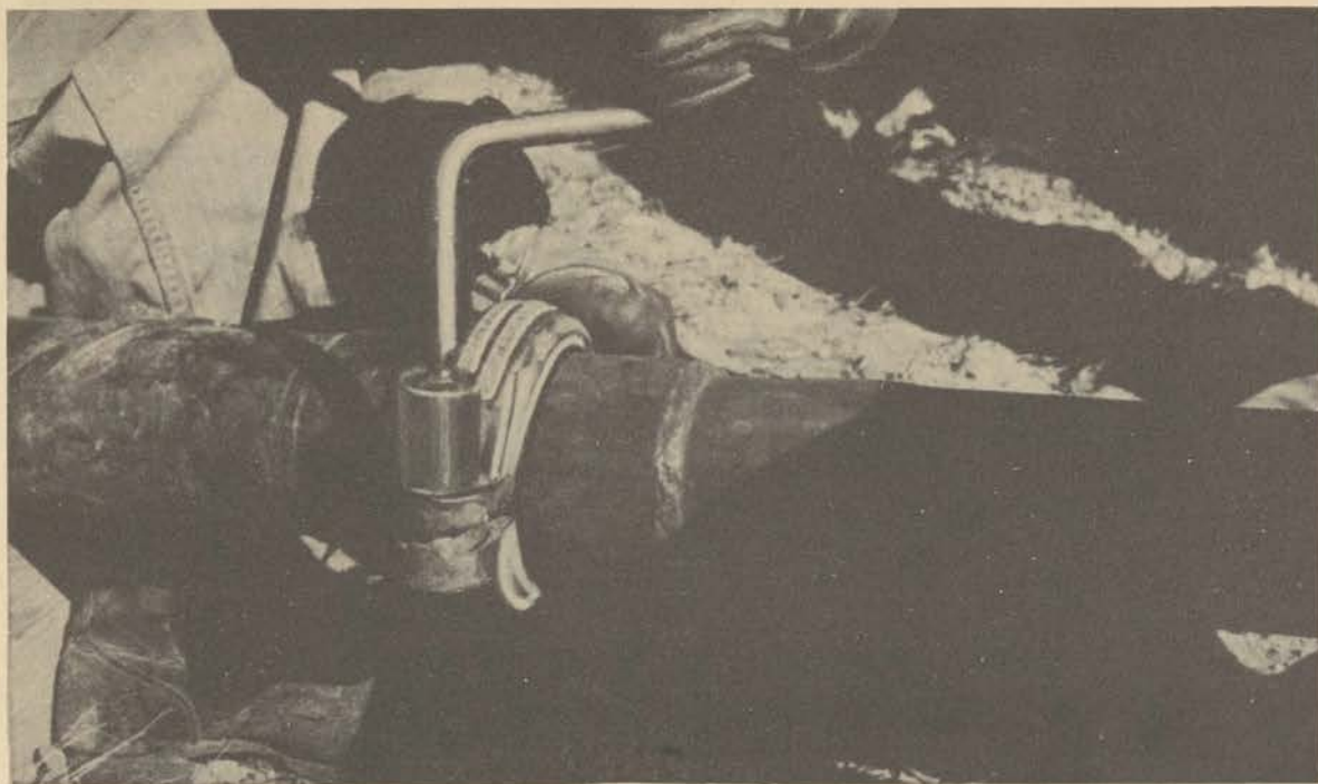
Figure 57. Turning the nuts down evenly.
