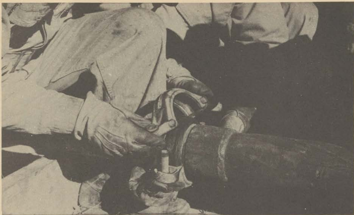
Figure 55. Placing bottom and top halves of coupling over the gasket
