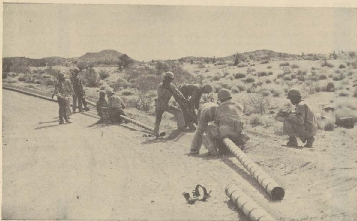
Figure 48. Two four-man crews connecting pipe.
