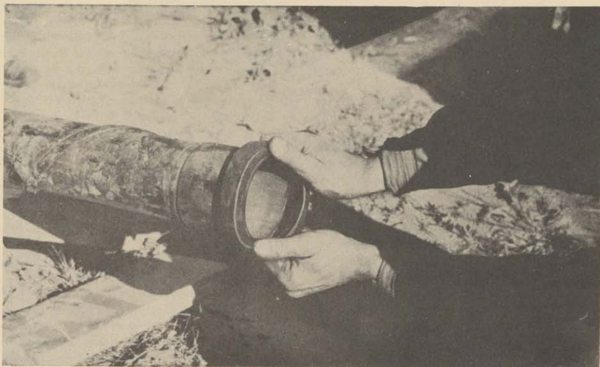
Figure 51. Placing gasket on pipe end.
