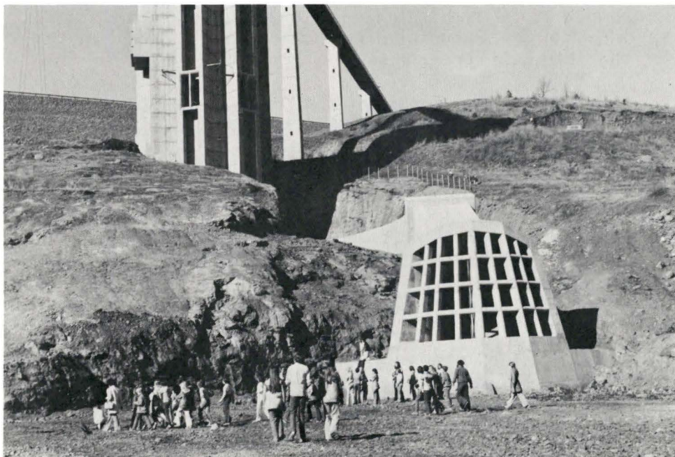
Intake for the turbidity conduit at Lost Creek Dam
