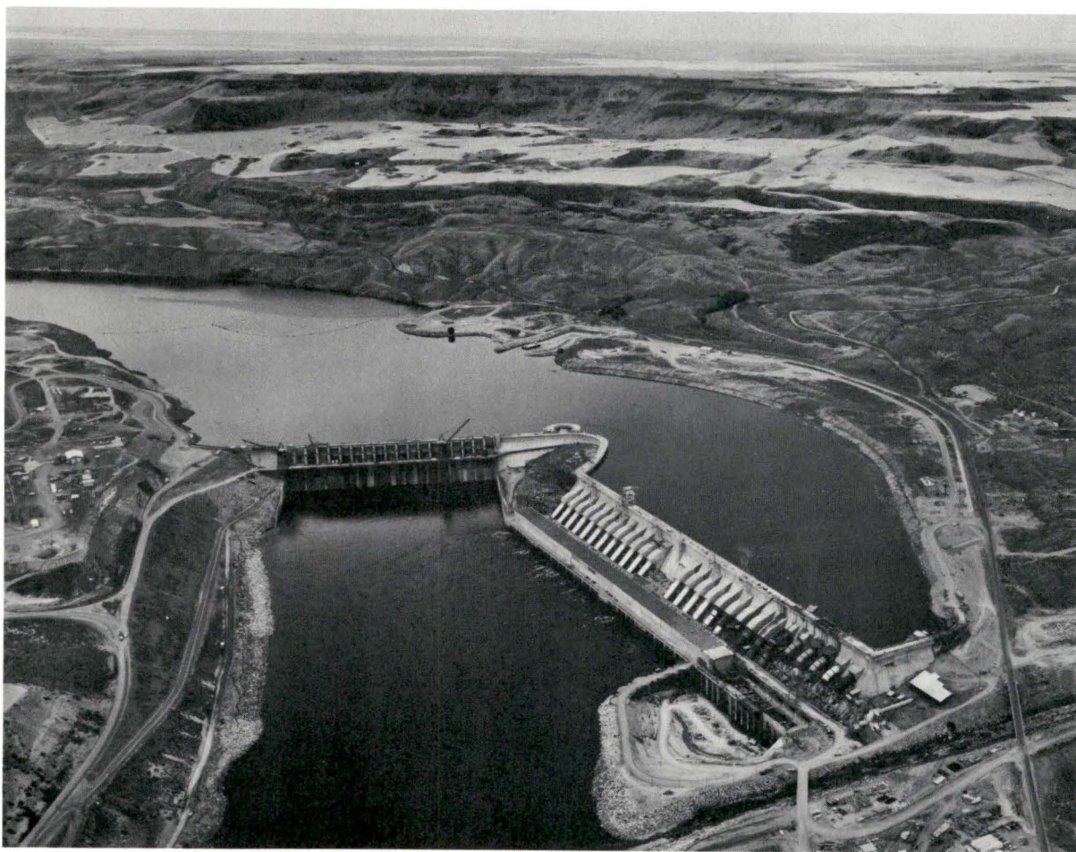
A July 1977 view of Chief Joseph project showing construction of the spillway modification and eleven additional generating units. The modification will increase the normal maximum pool elevation and add 1,045,000 kilowatts to the name plate rating of the project.
