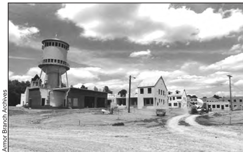
Figure 108. The mounted urban training site built at Fort Knox to support the training of heavy forces in built-up areas.
