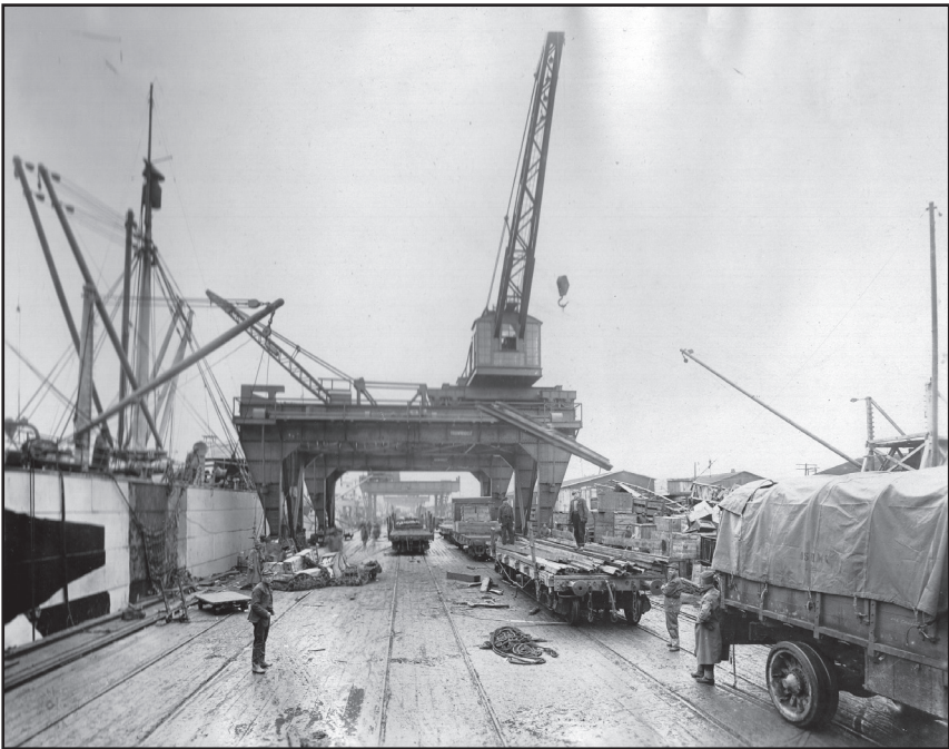
Figure 3.2 Once installed, the gantry cranes at the American-constructed port in Bassens significantly increased the efficiency of the cargo operations. Photo courtesy of the US Army Quartermaster Museum.
