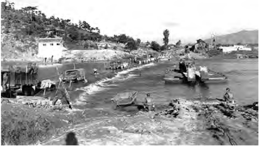
A river crossing via an underwater bridge (left) and a makeshift ferry (National Archives)
