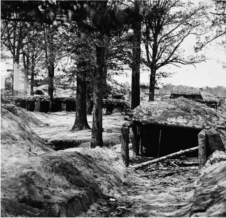
Interior of Fort Stedman (Library of Congress)
