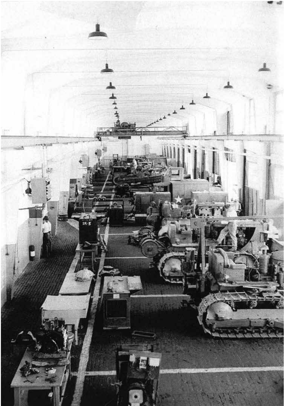
Field maintenance shop in Rheinau, Germany, 1959
