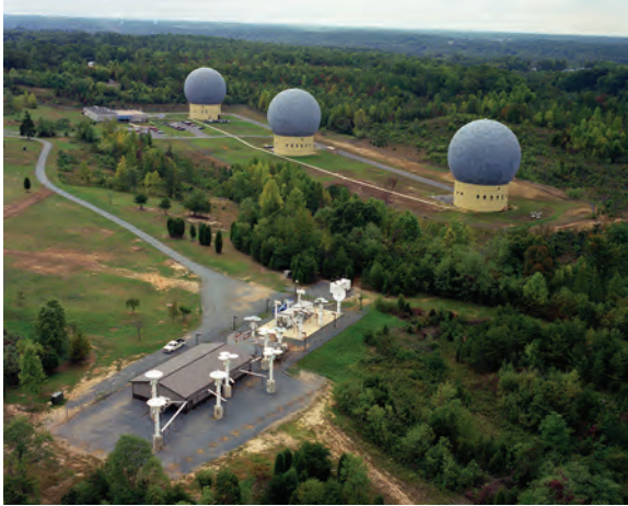
Midway Research Center. The three 18.2-meter-diameter tracking antennas at NCST's Midway Research Center, located in Stafford County, Virginia (and with associated tracking facilities in Palo Alto, Guam, and elsewhere), can transmit precision test and standardization signals to on-orbit satellites for such jobs as performance validation and verification, calibration, and anomaly identification and resolution. MRC also hosts an Optical Test Facility, built several years after this 1997 photo, for developing optical communications techniques and ground-to-air laser-based tracking capabilities. (NRL photo 98-000006(16).jpg)
