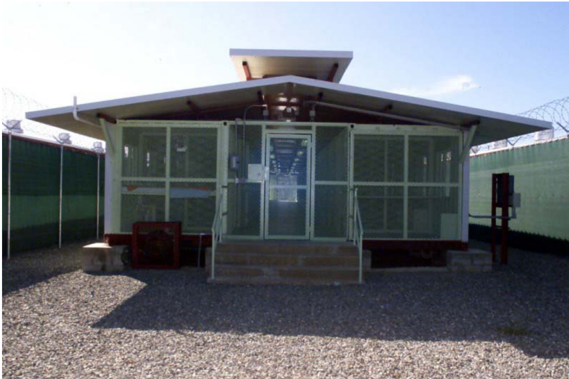
Long-Term Detention facility
