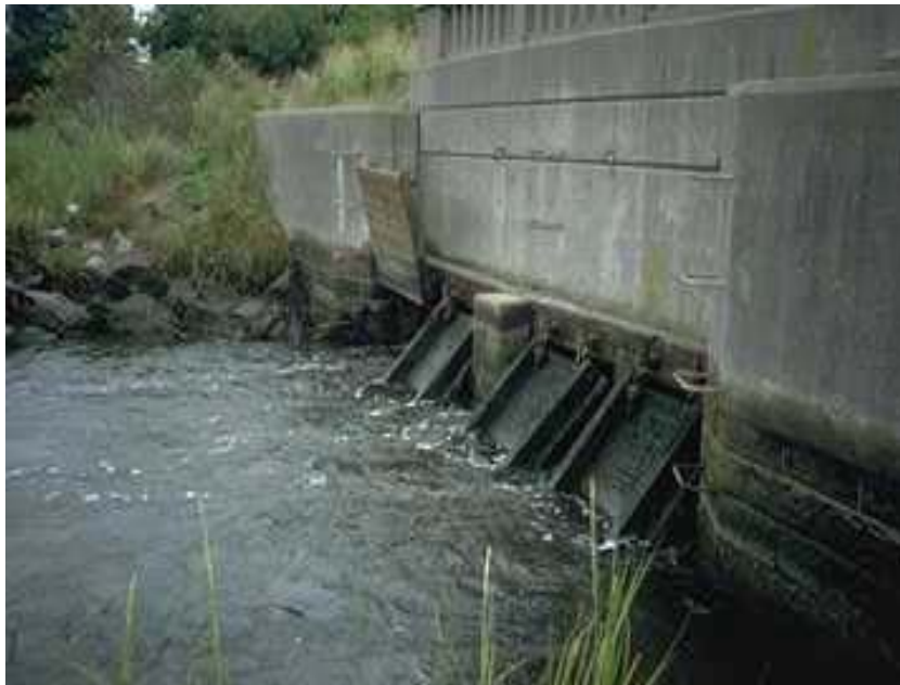
FIGURE 1-3. One of Four Flap Tide Gates Open at Hammock River
