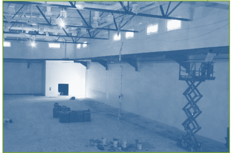
Workers construct the track inside SKC's health and fitness center.
