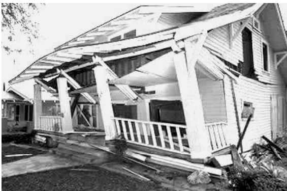
Figure 3 - Northridge Earthquake, Jan. 17, 1994 Single-family residence damaged due to failure of multiple elements.
