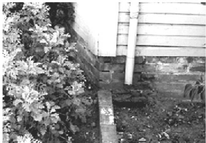
Figure 17 - Note the bricks exposed in this unreinforced masonry foundation.
