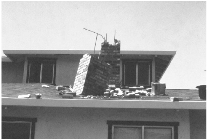
Figure 30 - Morgan Hill Earthquake. Broken chimney fell on roof.
