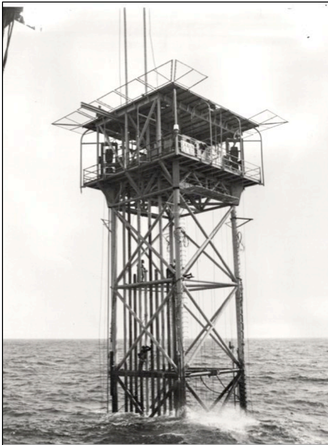
Figure 1.9. Exxon's 1/50 scale guyed tower test model, pictured December 1975 in Grand Isle 86
