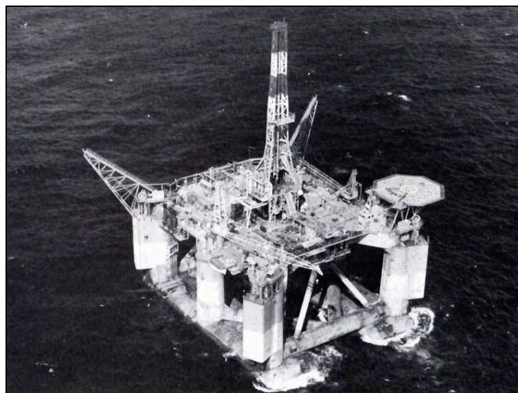
Figure 1.1. The Penrod 72 semi-submersible drilling rig, circa 1988, after conversion to a production unit for use at Green Canyon 29
