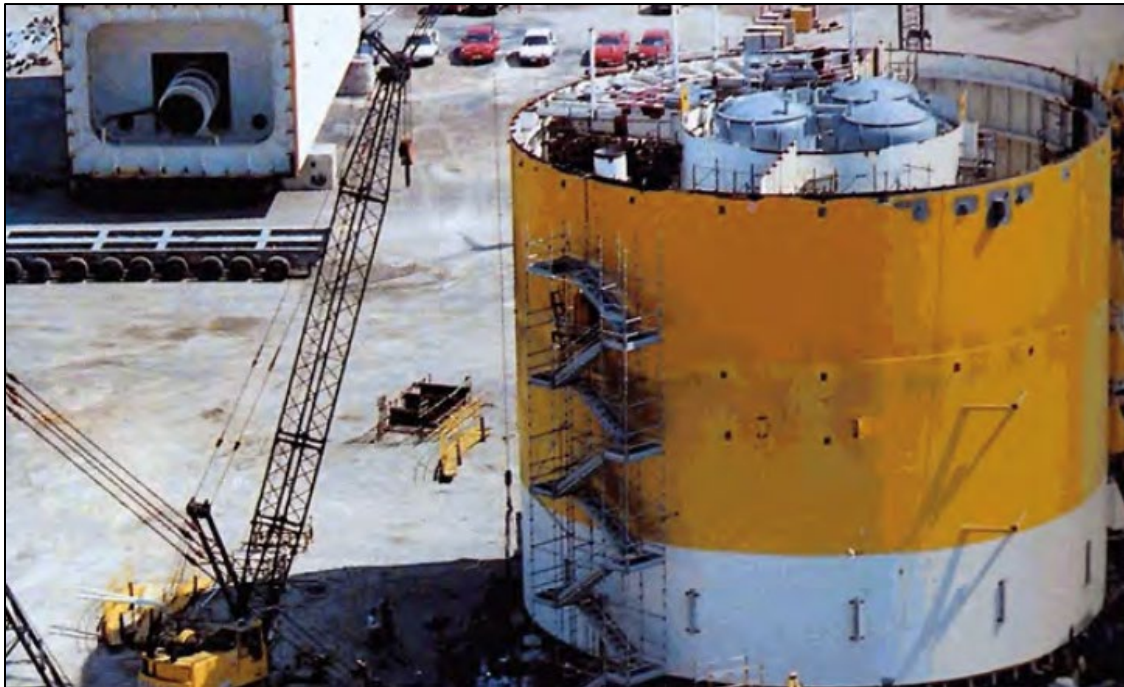
Figure 1.23. One of four columns fabricated by Belleli S.p.A. for Shell Oil’s Auger tension-leg platform
