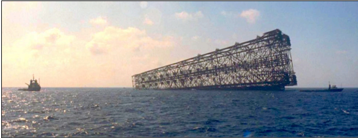
Figure 1.22. Shell's Bullwinkle jacket is towed out to its installation site in the Green Canyon right before its launch in 1988
