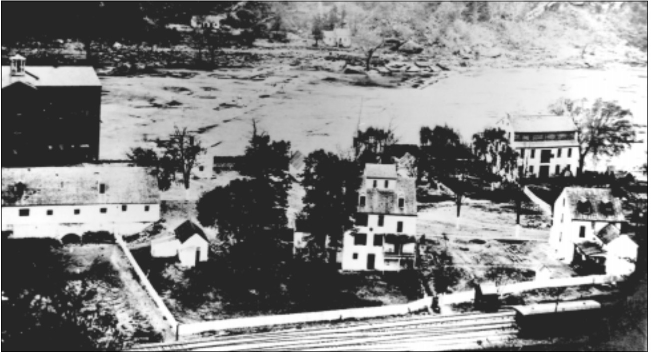
Figure 1. This photograph of Virginius Island shows the proximity of the former industrial community to the Shenandoah River. The nineteenth century buildings were largely destroyed by successive floods by the turn of the century. A geophysical survey of selected areas of the island yielded information about the location of ruined residences and outbuildings. This information was used in developing a treatment plan for the cultural landscape. Harpers Ferry National Historical Park. (NPS, 1865)
