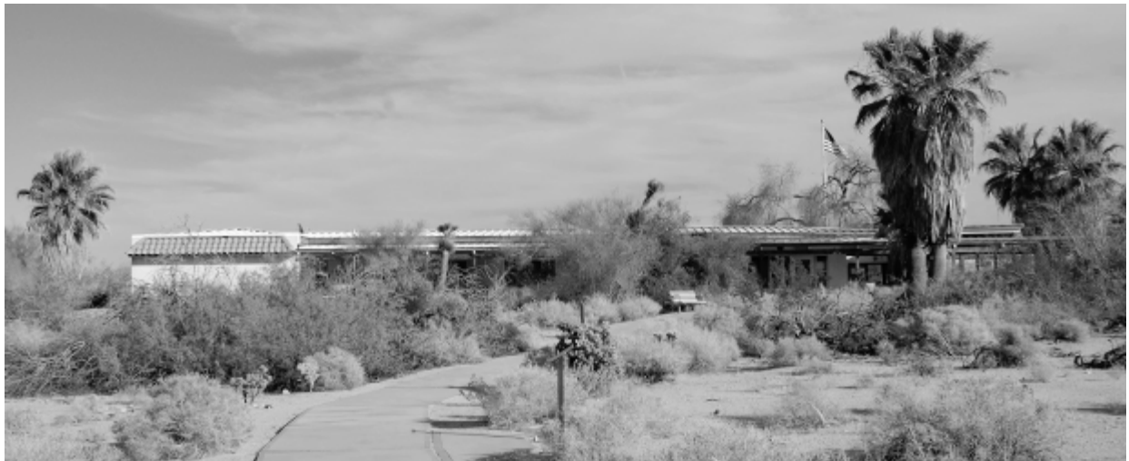
Figure 6-2. One of the Park Service's most influential architects, Cecil Doty, designed the Joshua Tree National Park Visitor Center, a classic example of Mission 66 architecture completed in 1963. The author took this photo from the nature trail through the Oasis of Mara.
