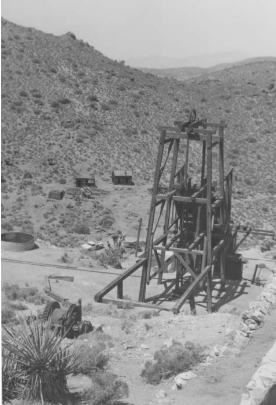
Figure 6-7. The Lost Horse Mine in 1967 before the headframe collapsed. The mine has suffered dangerous deterioration below the surface as well. Photo by Donald Black. JTNP photo archives, Cat. 20575, Image 1370.
