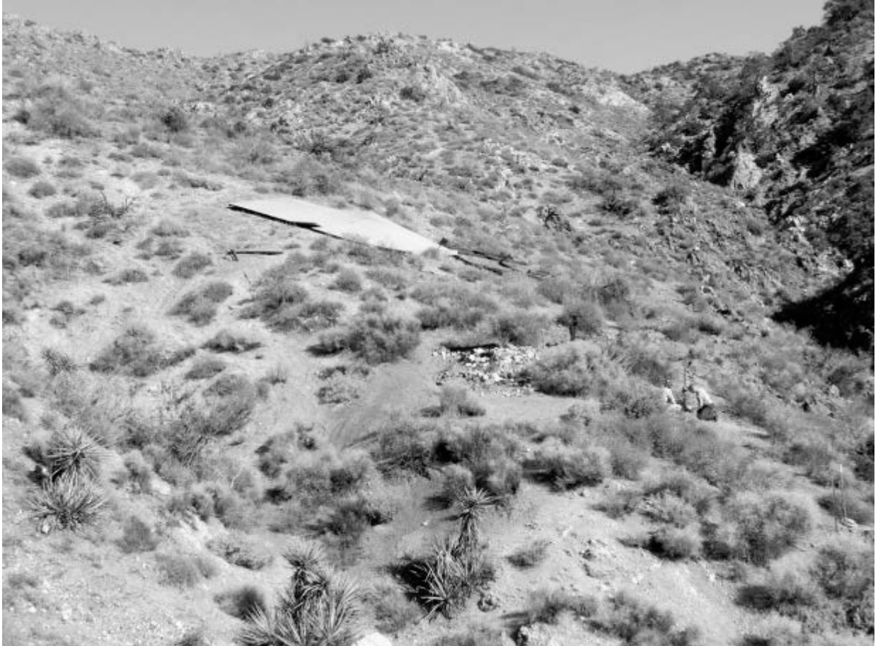
Figure 6-4. A guzzler consists of a broad rock face or piece of sheet metal that directs precipitation or piped water to a tank or trough. Downhill from the metal sheet two Park Service employees conduct repairs. Photographer unknown. JTNP Natural Resource Division files.
