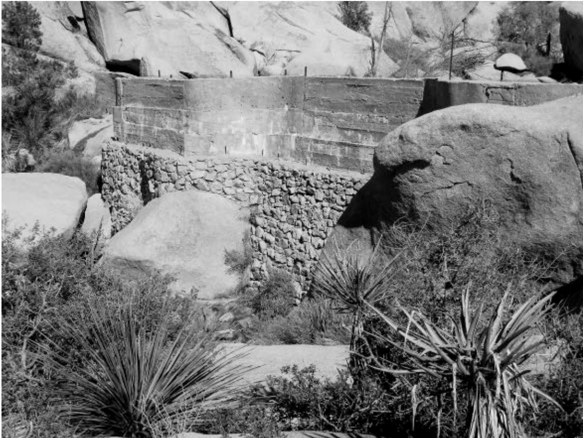
Figure 5-1. Barker Dam showing the original portion built by cattleman C. O. Barker and the upper portion added by Bill Keys. Photo by the author.
