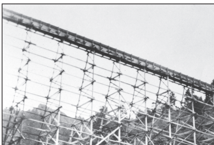
Flume and trestle over the East Fork of Mule Creek c. 1910
