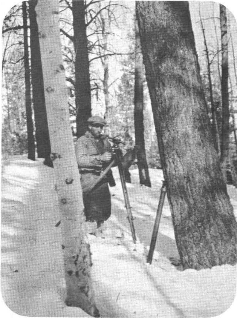
Survey of the 9th Standard Parallel North, T. 37 N., R. 2 E., Gila and Salt River Meridian, Arizona, November 1925. William E. Hiester, U.S. surveyor, at the transit.
