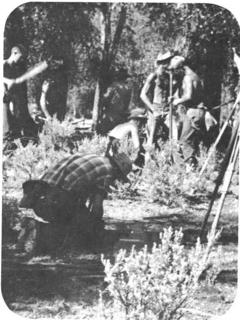
August 26, 1948, on the Utah-Wyoming State line near mile post 37. The survey party is under the direction of F. Wayne Forrest. The man in the foreground (kneeling) is stamping the section number into the brass cap of a survey monument.
