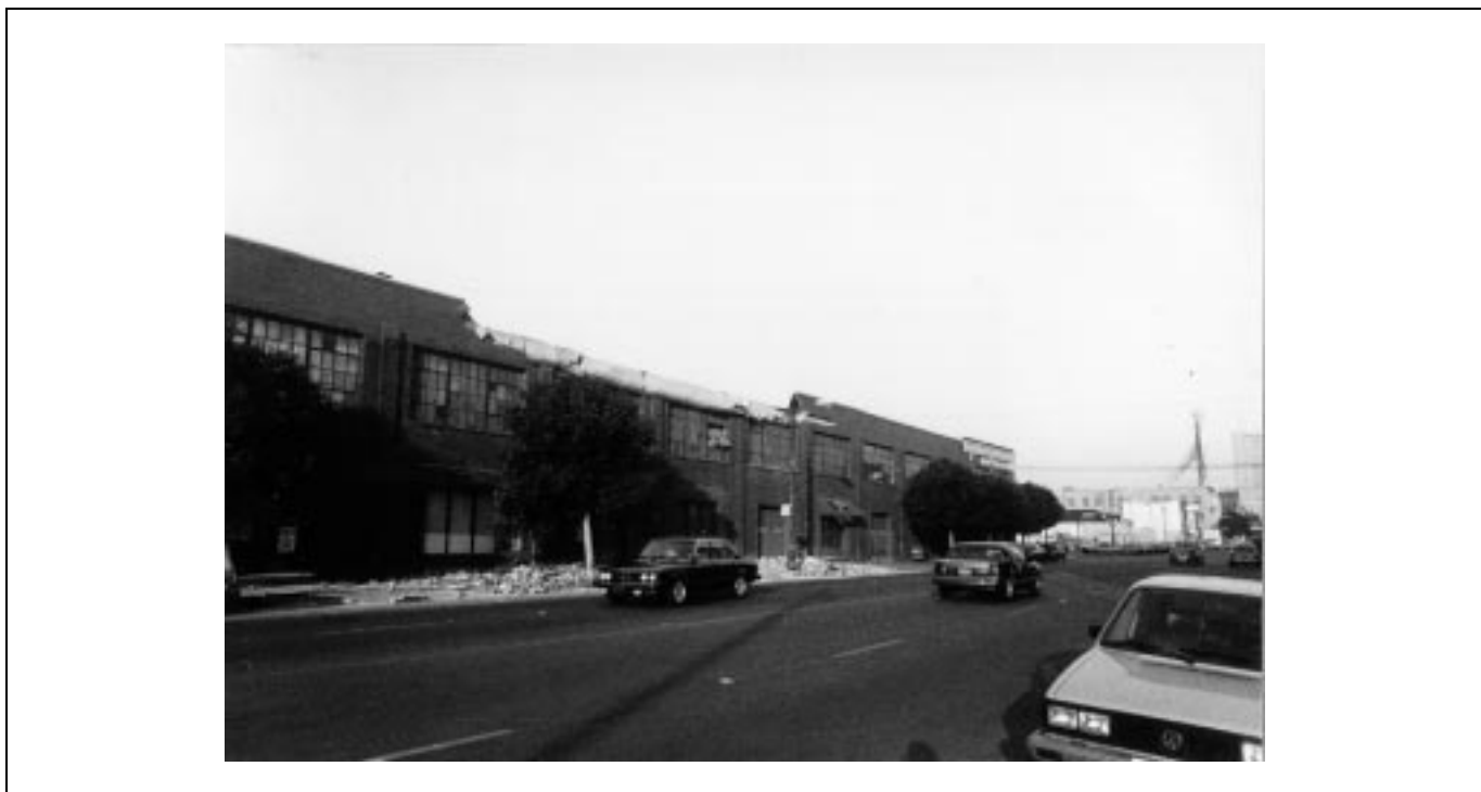
Figure 7-2 Photo of Parapet Failure (from Rutherford and Chekene, 1990).
