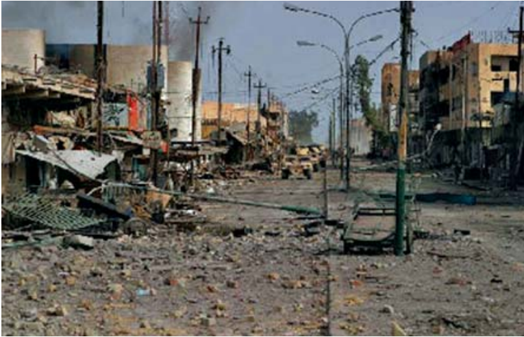
Condition of the city streets in Falluja in November 2004. (USACE photo)
