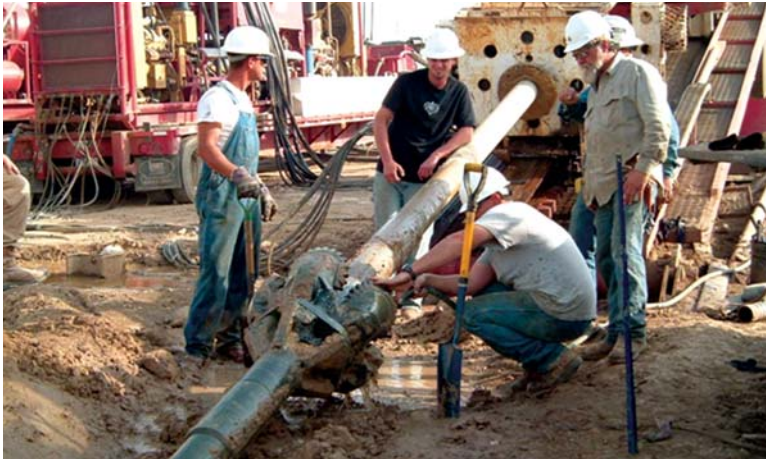
HDD rig with backreamer.
