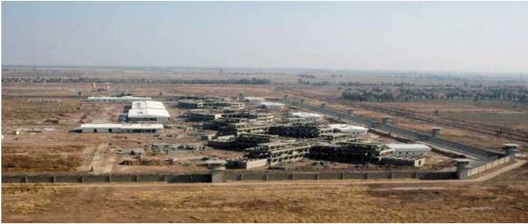
Kahn Bani Sa'ad Correctional Facility. (USACE photo)
