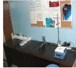
WTP laboratory equipment inventory did not include items necessary for performing jar tests.
